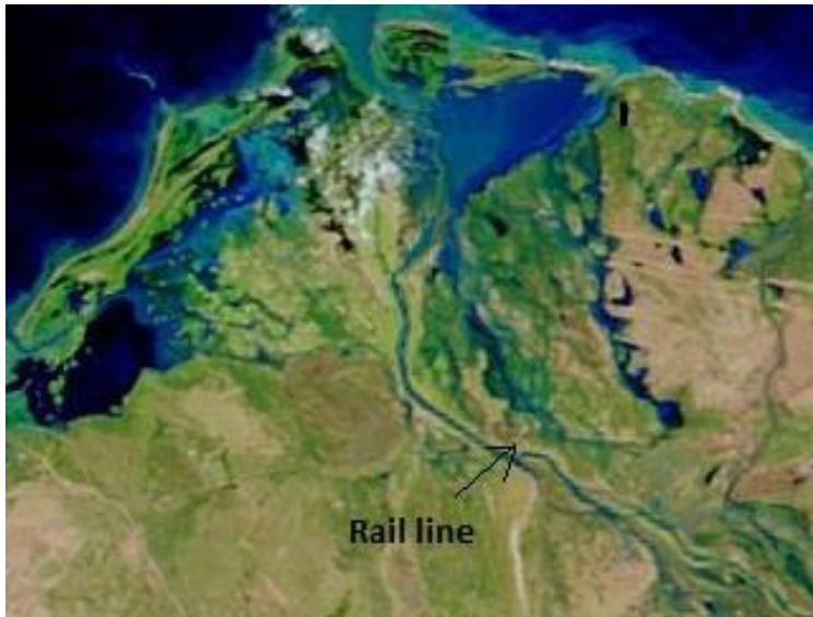
Figure 28: Water flowing on to the flood plain after the BHP Billiton rail failed from Cyclone Rusty flood waters.
