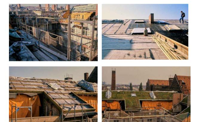
**Figure 2.** Details of the green roof installation in September 1985. Upper row: Scaffolding and lifting the older roof to construct the roof level apartments. Lower row: Installation of the thrust-thresholds and the PVC layer. Lower right: With the final turf mat layer.
