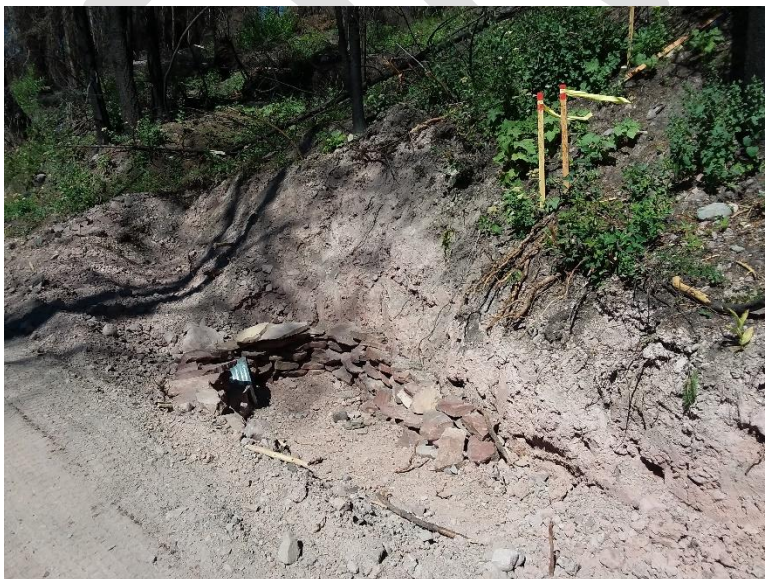
Photo 2: Culvert located at a GRHO sub-population site
