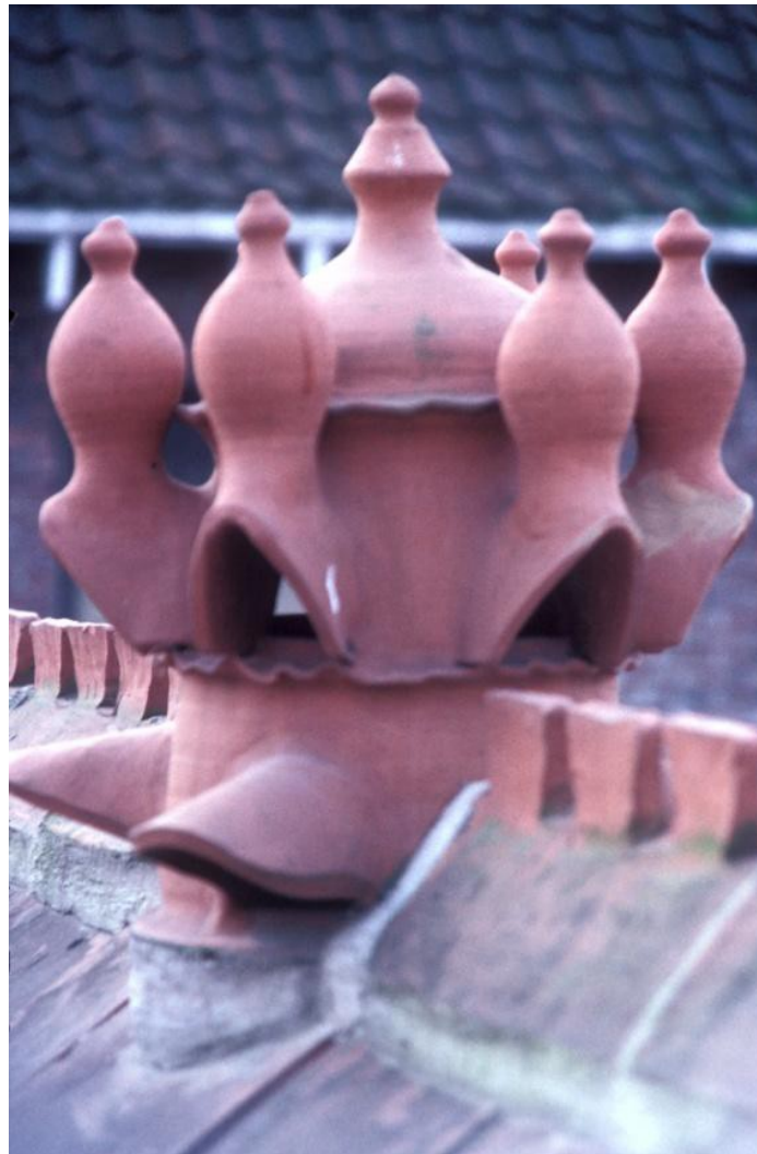
Plate 23: A replica medieval louver on the roof of Barley Hall, York
