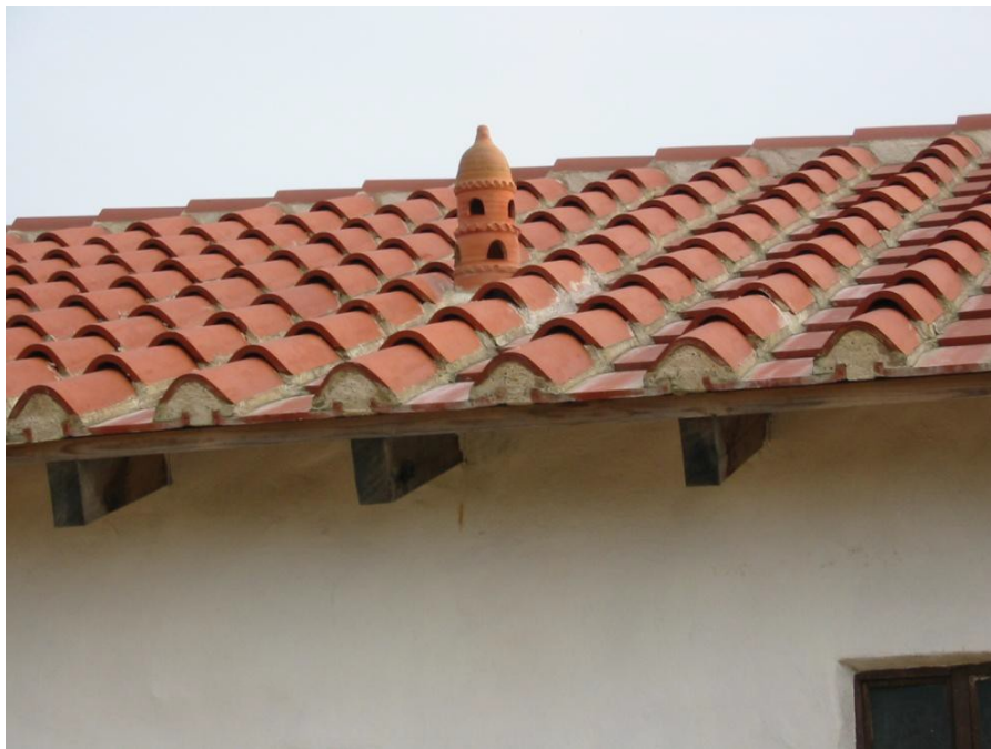
Plate 6: A reconstructed Roman roof of imbrices and tegulae at South Shields, South Tynesid
