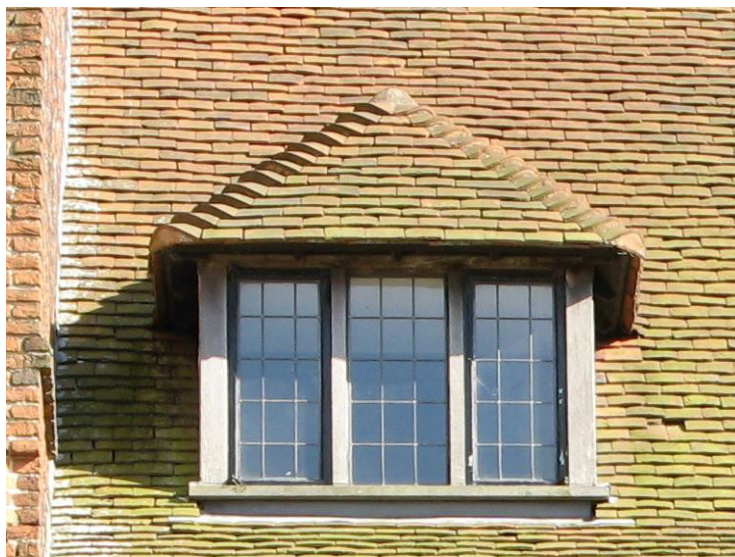
Plate 26: Hip tiles on the roof of Layer Marney Tower, Essex, which was built c.1520
