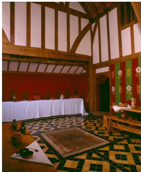
Plate 33: A replica plain glazed tile floor in Barley Hall, York
