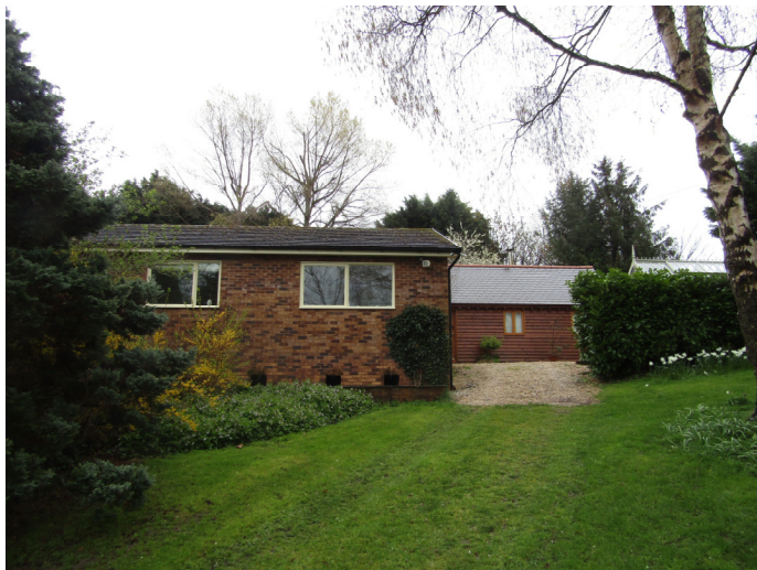
Photo 2: Existing dwelling and lodge [A6].
