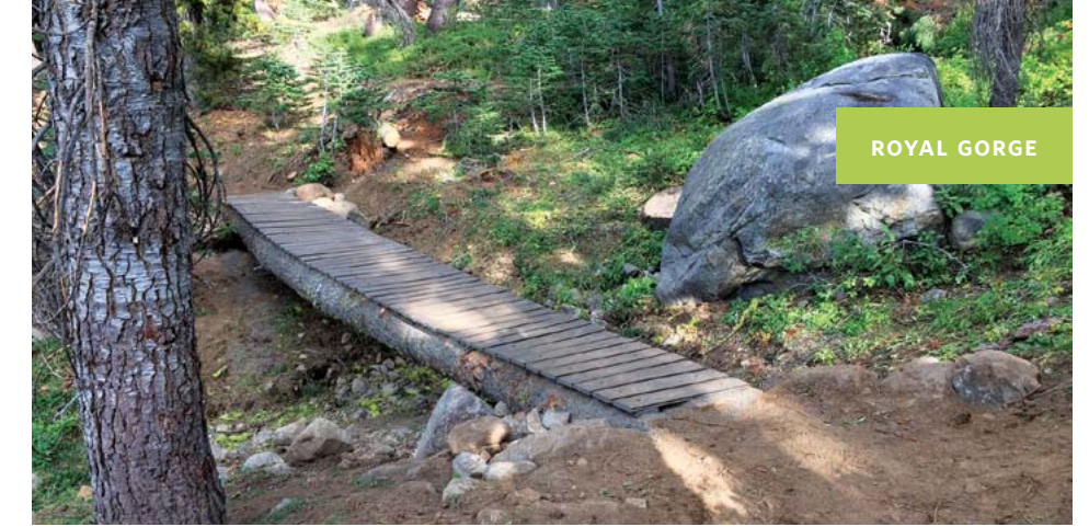
(left) Constructing a log-stringer bridge on the Walter and Esther Hewlett Rim Trail. (right) Voila, the finished product.
