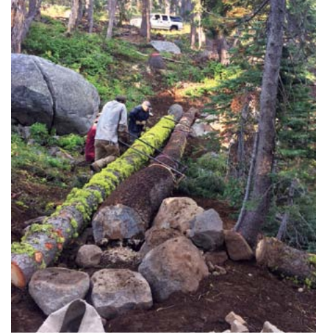
(left) Constructing a log-stringer bridge on the Walter and Esther Hewlett Rim Trail. (right) Voila, the finished product.
