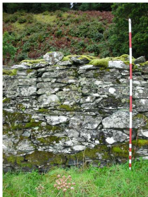
Structure 6 blocked window
