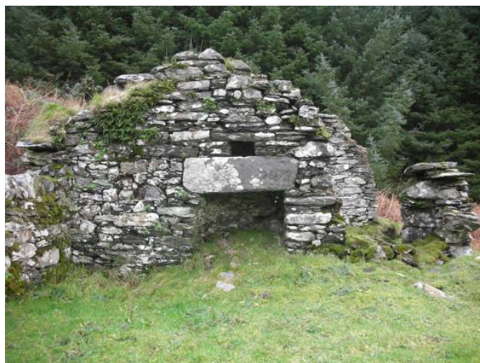
Structure 1 firepalce in north gable of central bay
