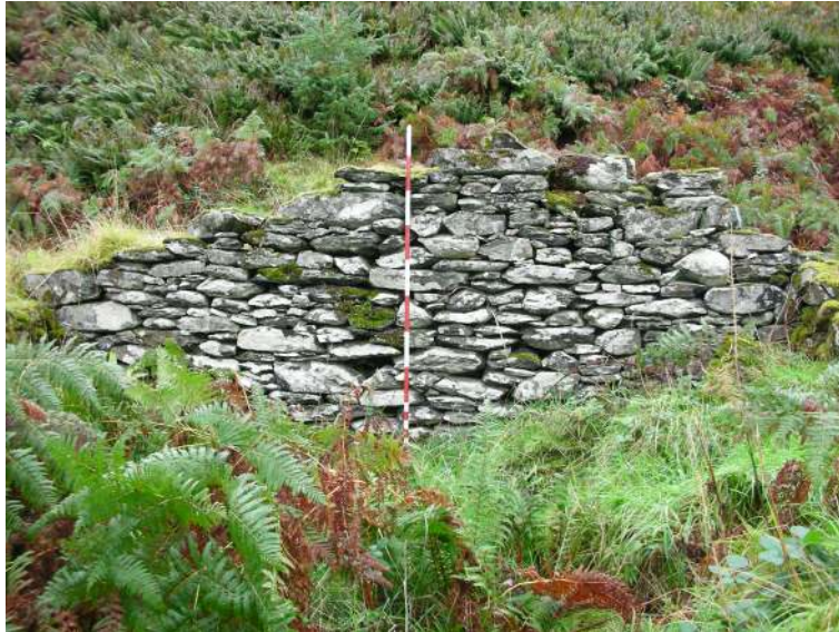
Structure 12 west gable
