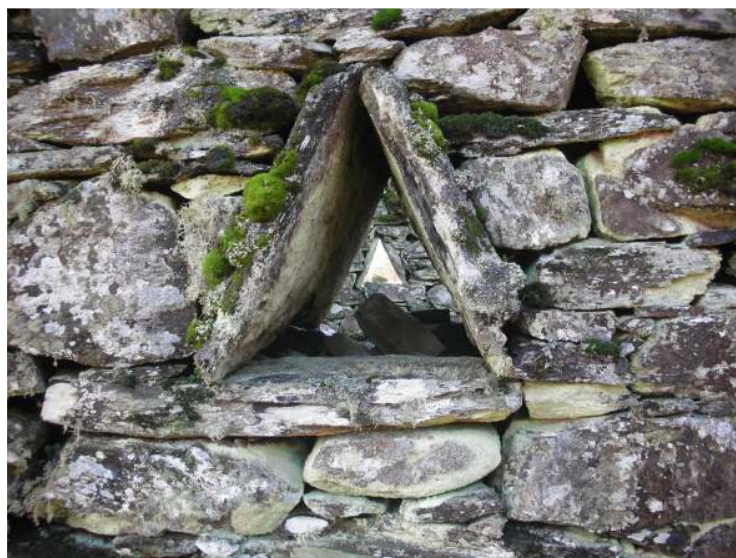
Structure 2 ventilation slots
