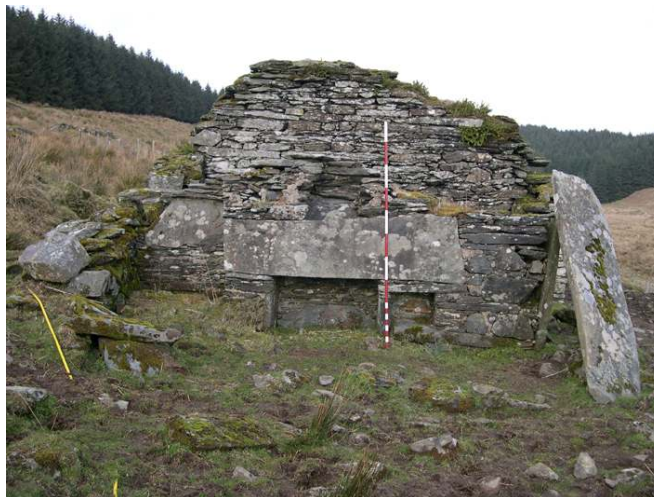
Partially demolished/robbed structure also at Leac na Ban
