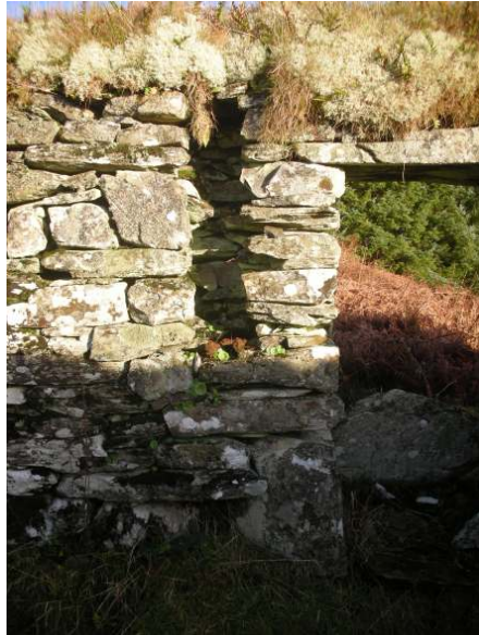
Structure 2 cruck slot
