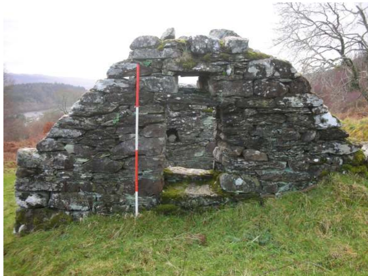
Structure 9 north gable
