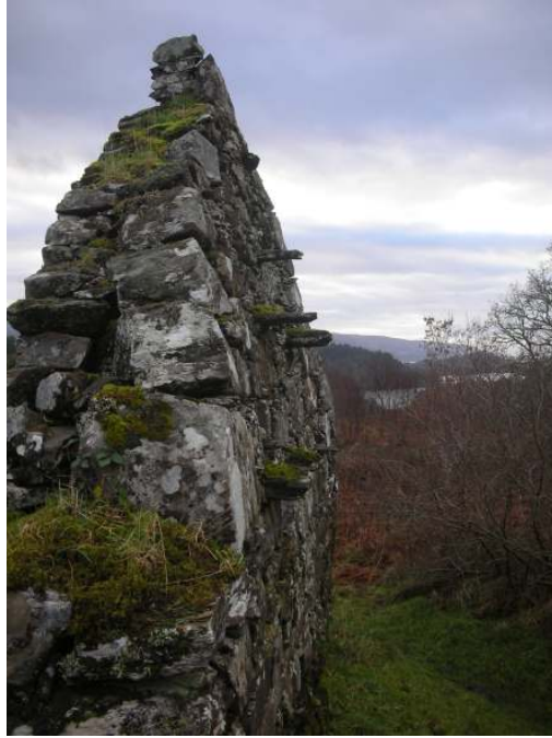
Structure 12 west gable
