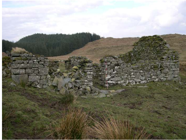
Barn structure at Leac na Ban
