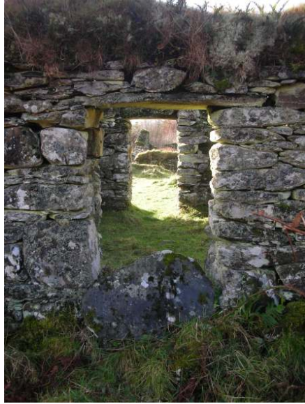
Structure 2 opposed doorways
