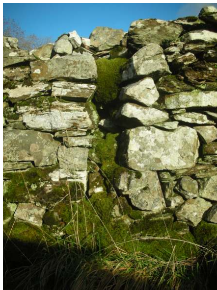
Structure 12 cruck slot
