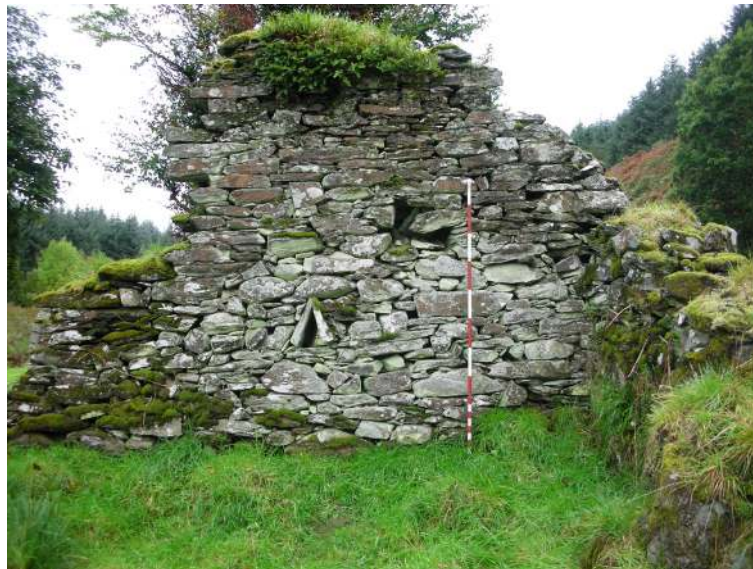
Structure 2 south gable internal elevation
