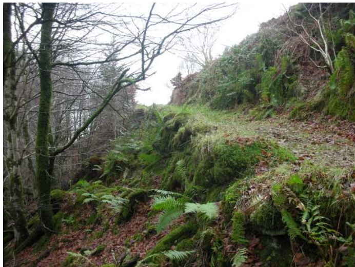
Stone revetting on track leading to Arichonan
