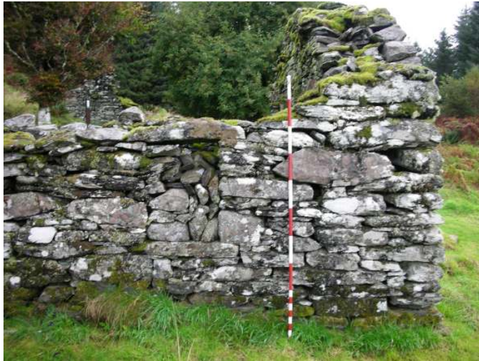
Structure 4 blocked window in south wall
