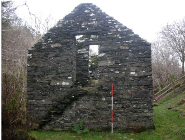
Southern side of mill structure
