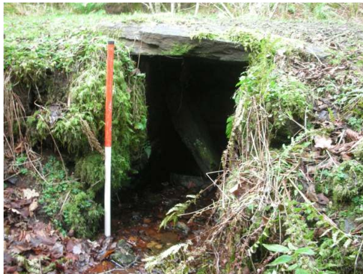
Stone lined culvert under present track
