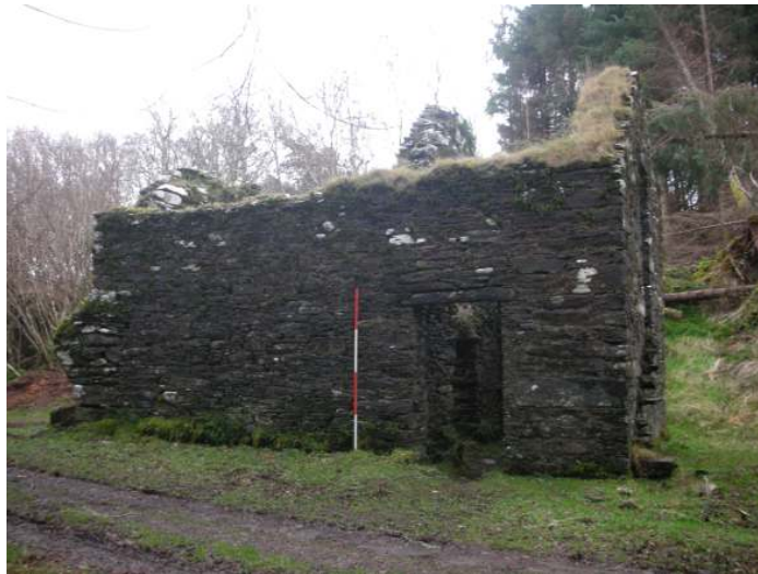
Western side of mill structure
