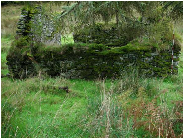
Structure 8 west side
