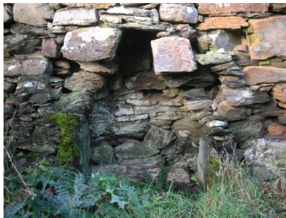
Structure 5 fireplace in west gable
