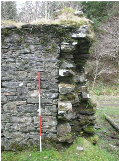
Junction of earlier and later stonework
