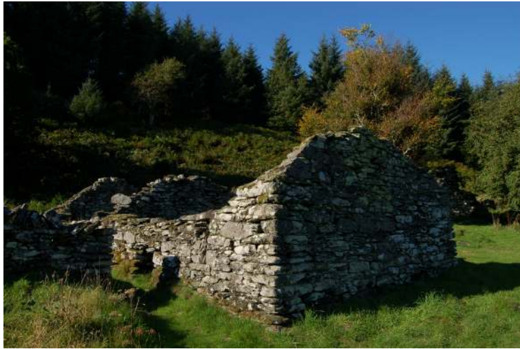
Structure 4 east end
