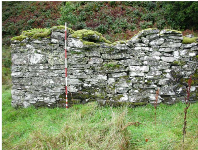
Structure 6 blocked doorway
