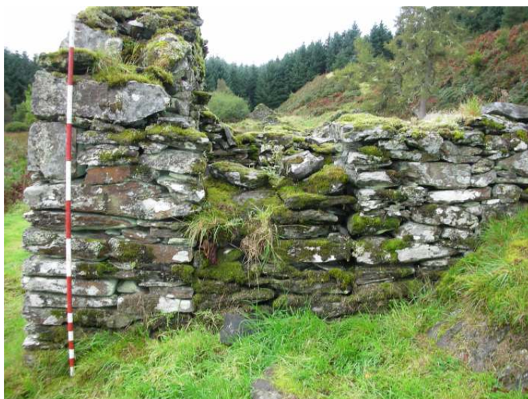
Structure 4 blocked door in north wall
