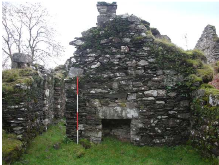
Structure 1 fireplace in south gable of central bay
