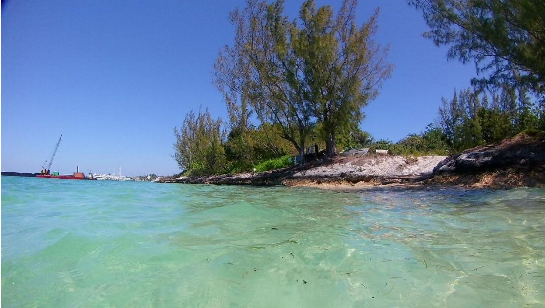
Photo 1: Rocky shoreline of the site with construction activities (view facing north)
