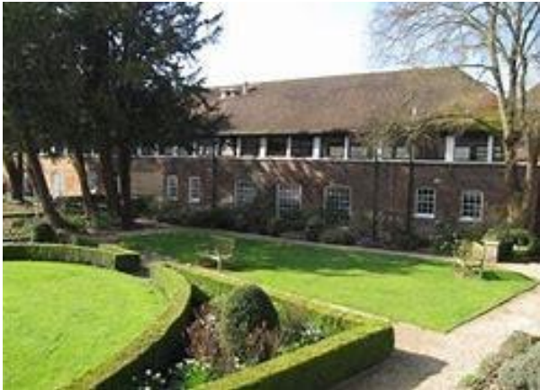
Figure 9 Turkey Mill Drying House as it is today. The interesting thing is how tastefully it has been converted to modern commercial use
