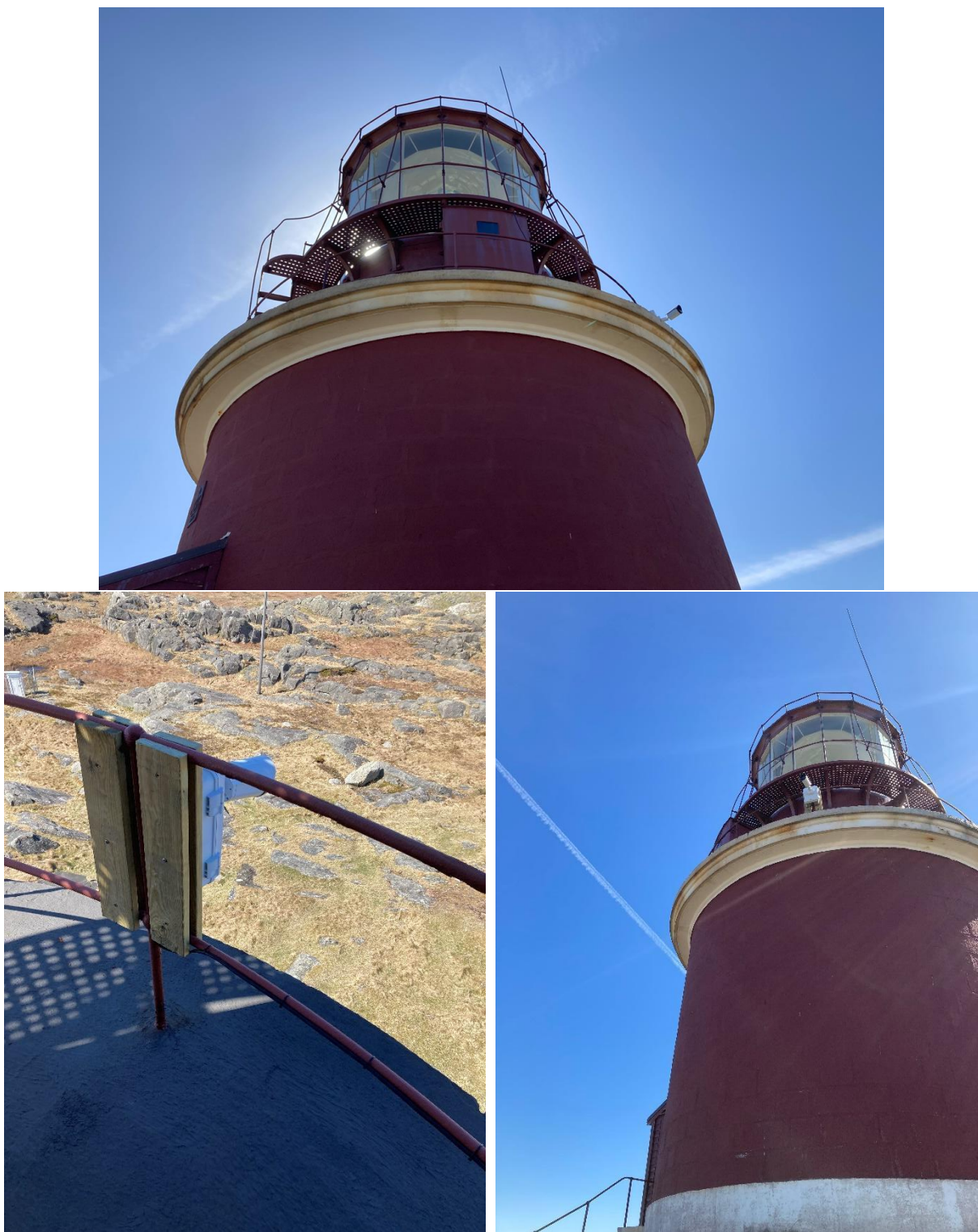
Figure 3: Installation on the Utsira lighthouse.
