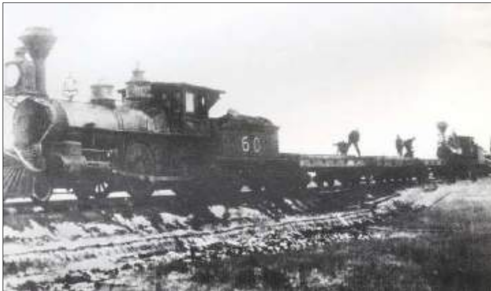
Laying track on CPR mainline – 1880s – (Source: PAS: _____) 158 kb
