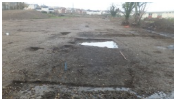
Fig. 6.38 Mid-excavation shot of the pond C243 and ditch C203, looking west
