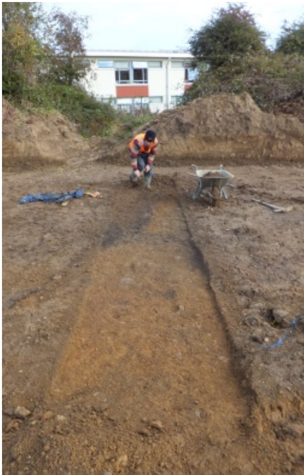
Fig. 6.19 Mid-excavation shot of spread C108 being removed with features visible beneath the spread
