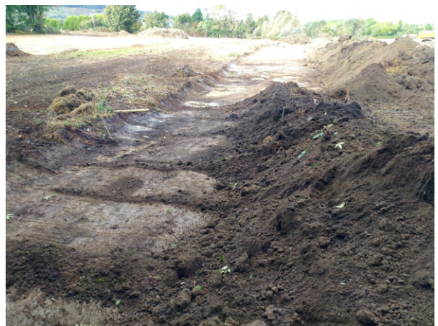
View of Area 2 after stripping, looking southwest (top)
