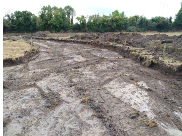
View of north-south road after stripping looking northwest (top)
