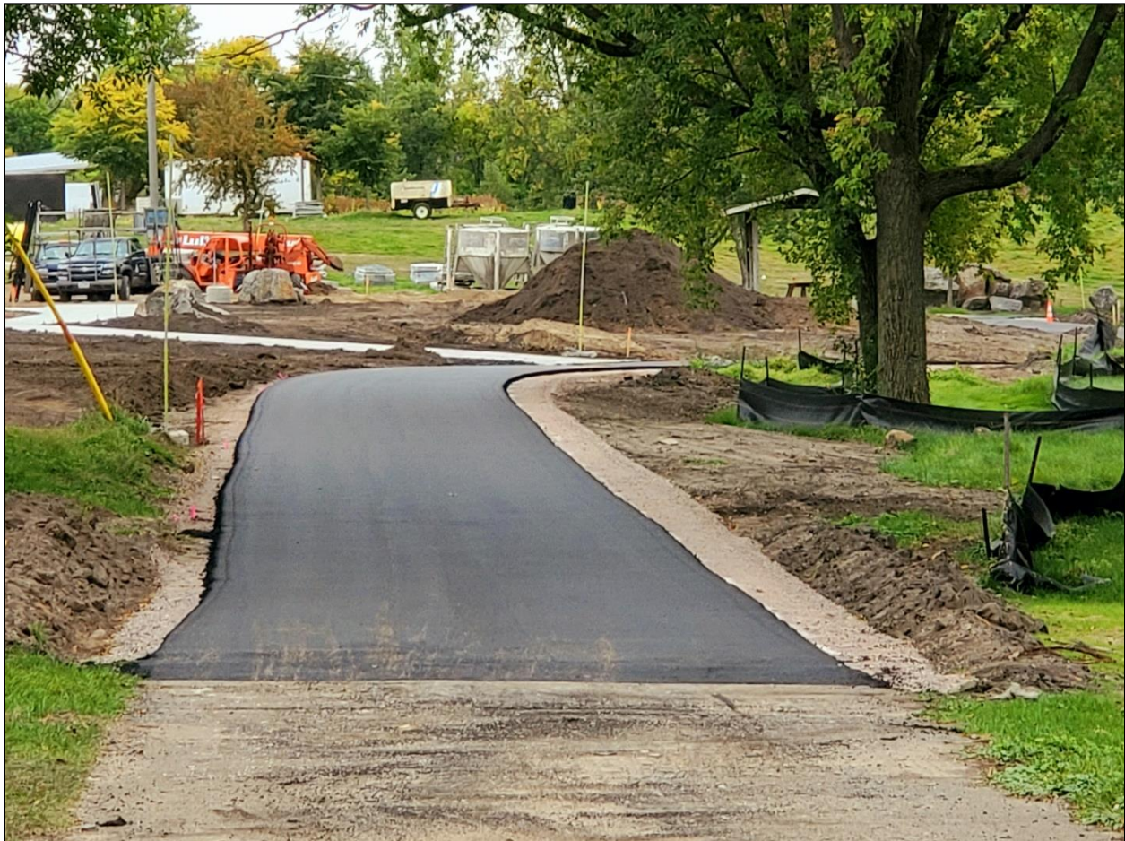
FIGURE A.11 - NEWLY PAVED SHARED USE PATH IN LIONS PARK.
