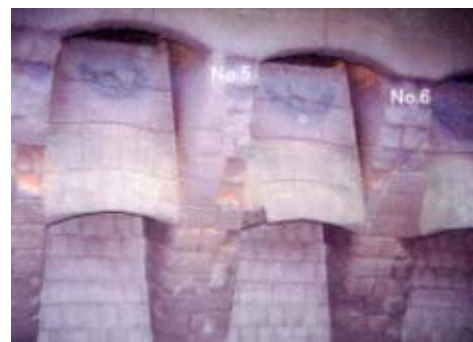
Figure-14 Photograph of refractory of Double flue after 5 years and 8 months operation (After change of the Refractory quality)
