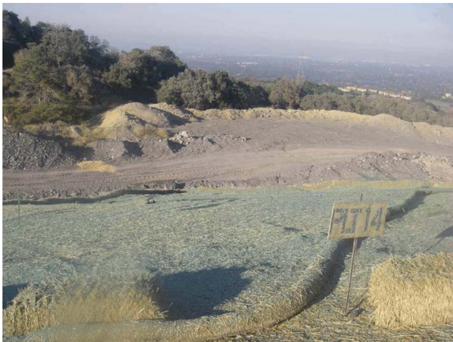
Top: Test Plot Construction: Applying Hydroseed Slurry at EMSA site.
