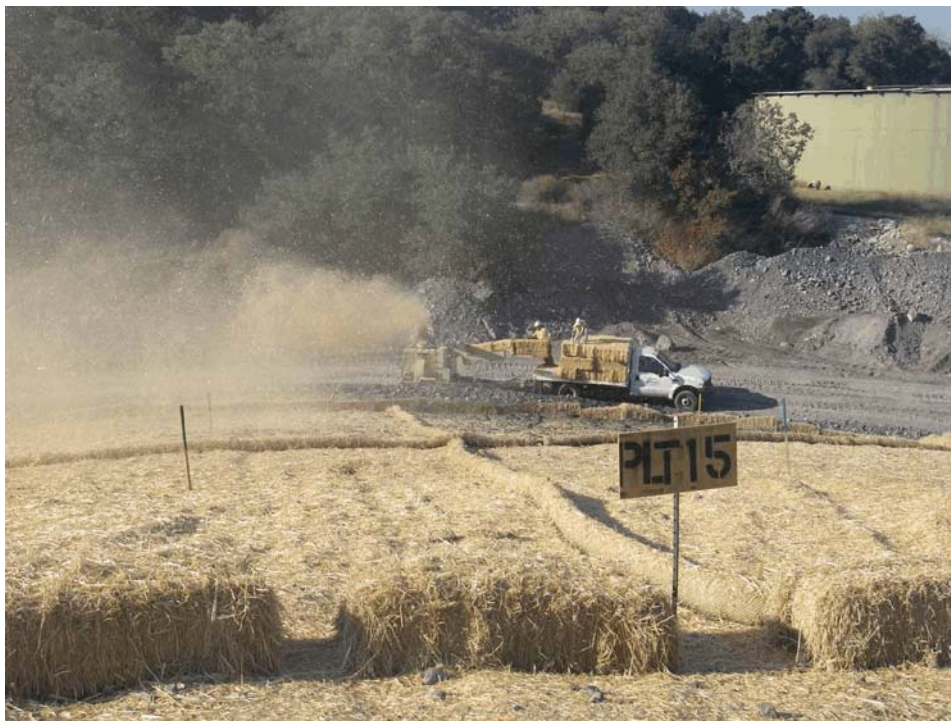
Top: Test Plot Construction: Applying Seed at the Yeager Yard site.
