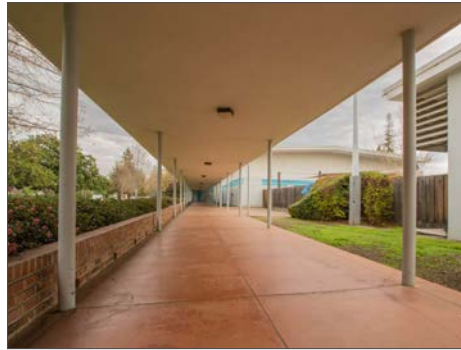
A | Outdoor covered walkways
