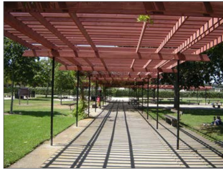
B | Pergola structure
