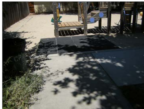
B | ADA access into play area
