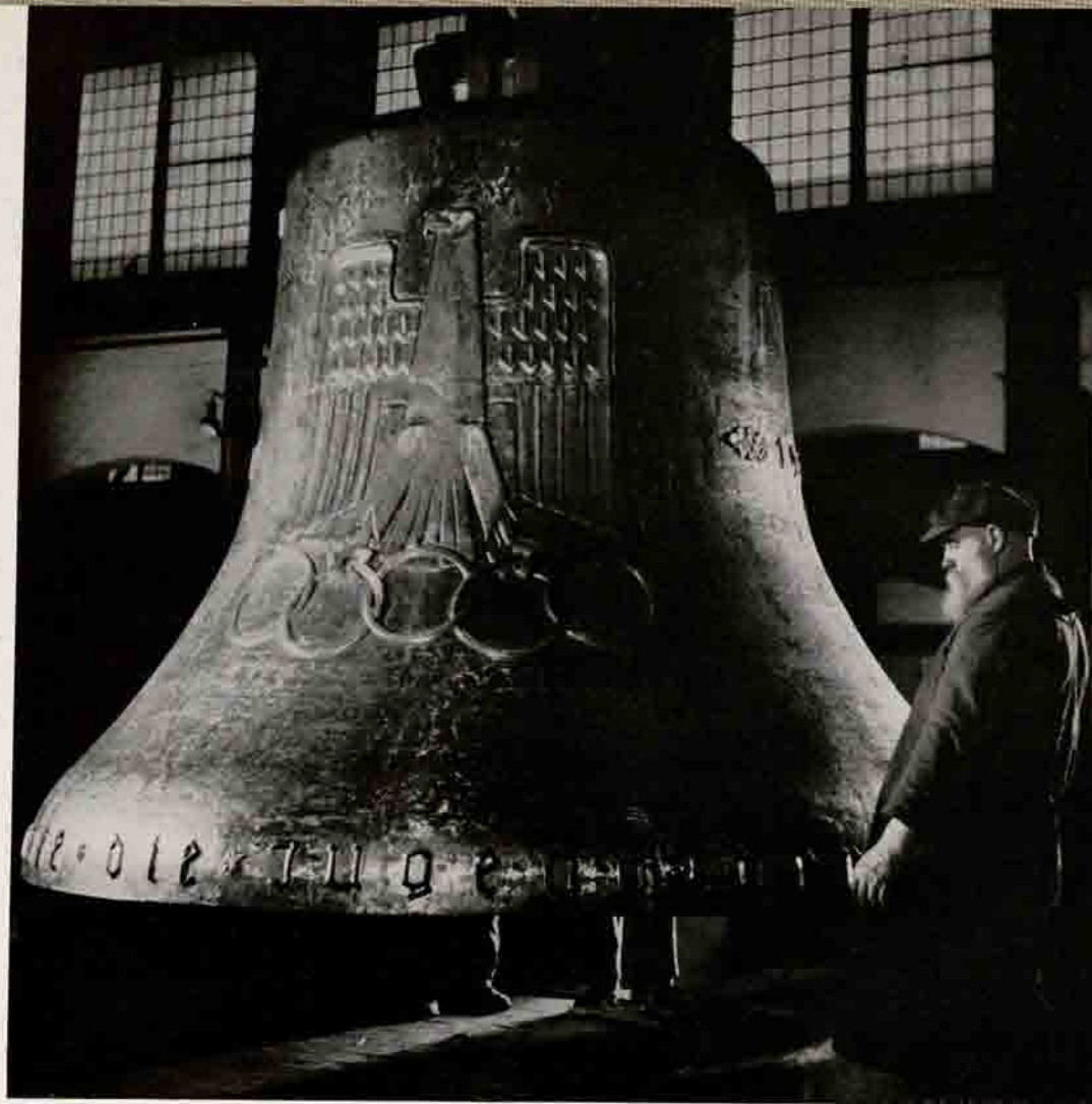
Cooling, polishing, chasing and tuning—and the Olympic Bell is completed.
