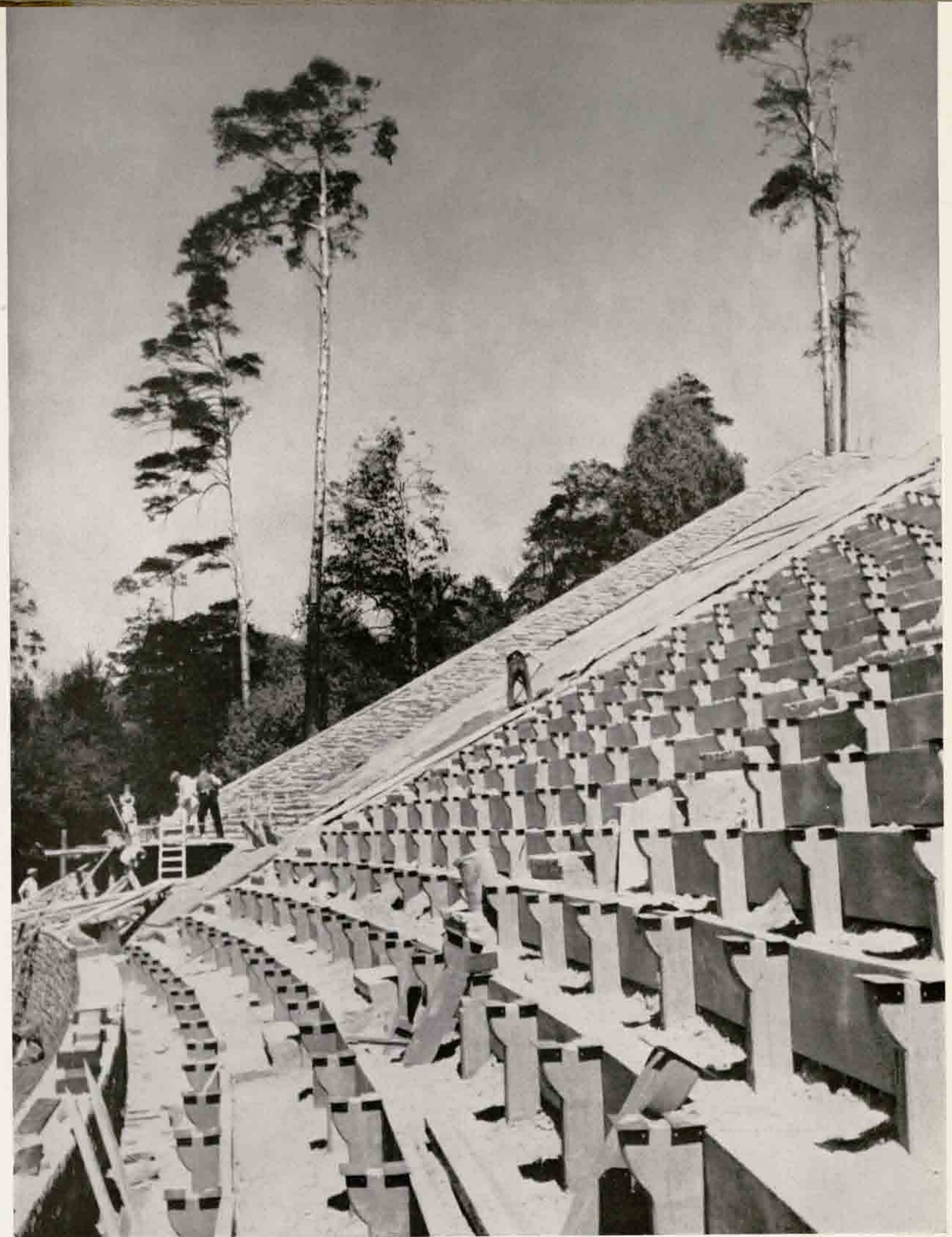
The Olympic amphitheatre, the Dietrich Eckart Open-Air Theatre, under construction.
