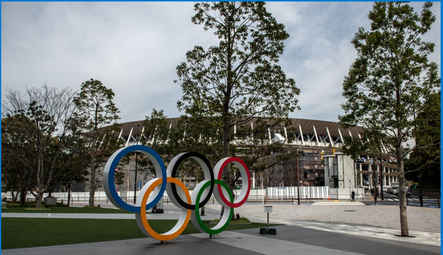
Tokyo's new Olympic Stadium has been constructed with multiple Dow technologies in paints, coatings, insulation and wiring
