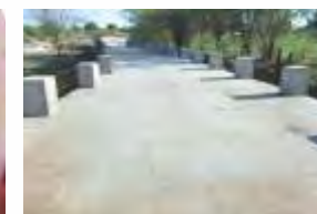
Construction of Roads
