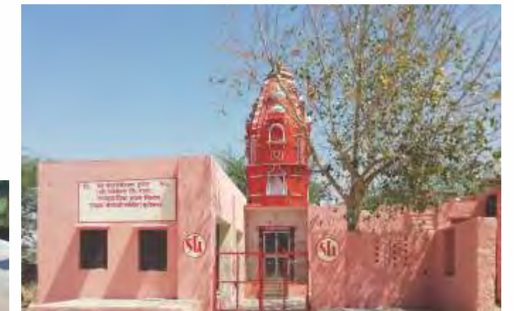
Community hall construction
