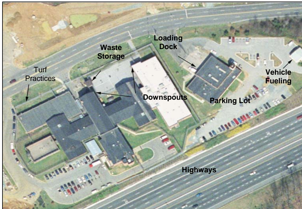
Figure 10: Operational Areas Subject to Infiltration
