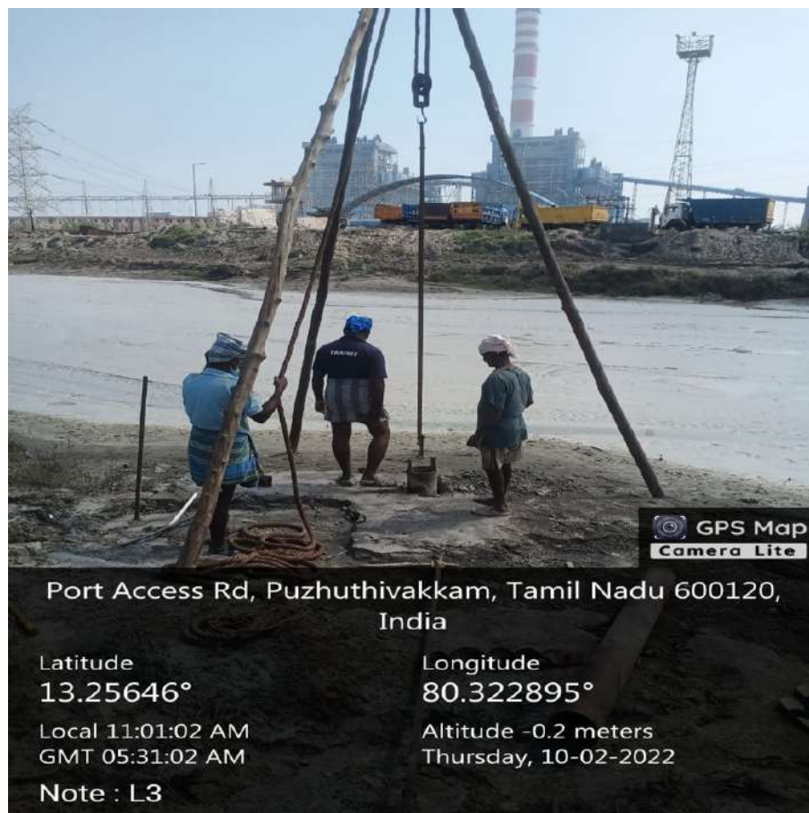
Figure 2 Deep drilling in the study area
