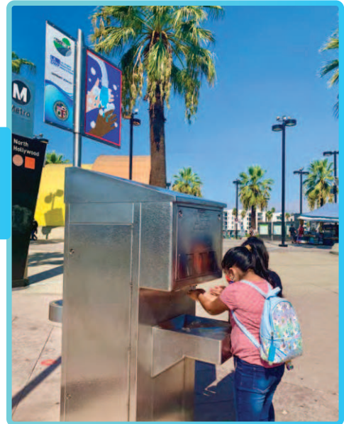
WORKING WITH StreetsLA, HAND-WASHING & HYDRATION STATIONS WERE INSTALLED TO MEET COMMUNITY PANDEMIC RELATED NEEDS
