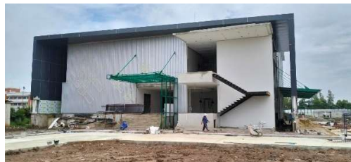
Tokamak Facility under construction
