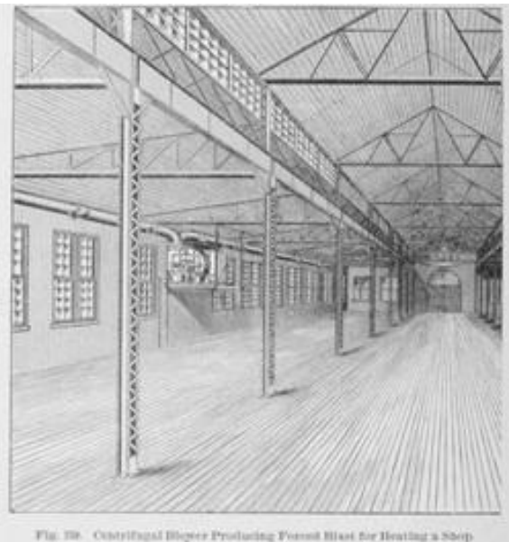
Fig. 138. Centrifugal Blower Producing Forced Heat for Heating a Shop.
