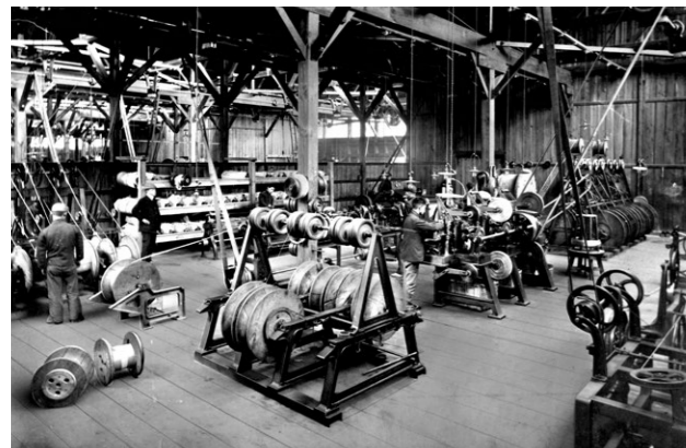
Copper Rolling Works Cable Plant (photo supplied by Sumitomo Historical Archives)
