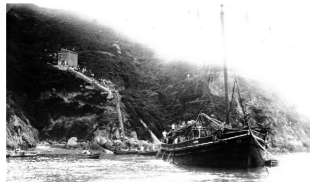
Landing of the cable end at Shisakajima on August 10
