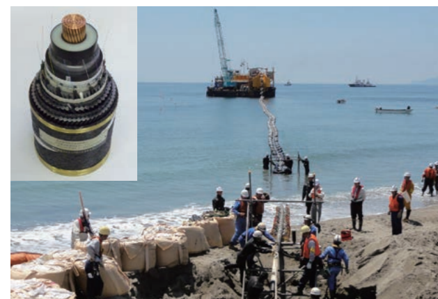
Construction of the Hokkaido-Honshu (Kitahon) HVDC Link
