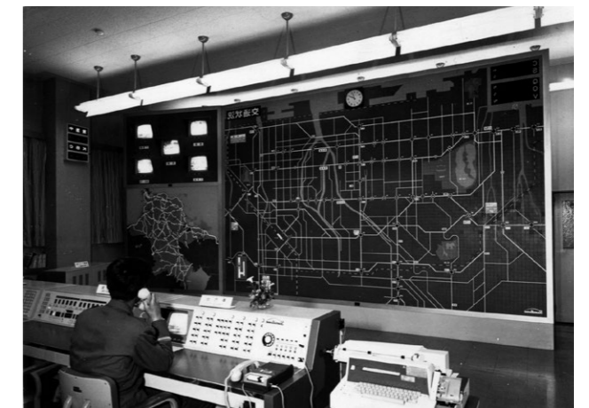
Japan's first wide-area traffic control system (Fukuoka Prefectural Police Headquarters)
