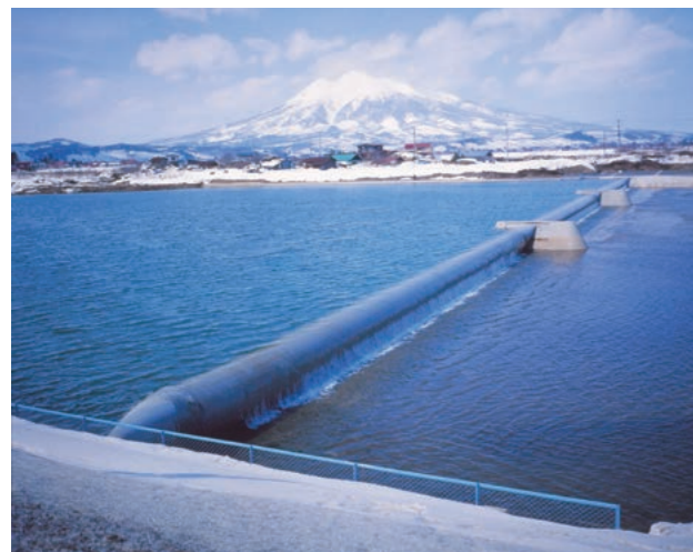
Iwakigawa intake weir Fabridam
