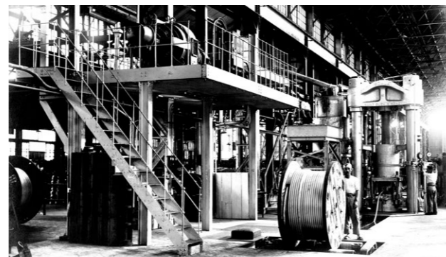
Lead sheathing machine at Sumitomo Electric Wire & Cable Works
