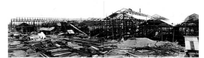
Construction of Okijima Plant
