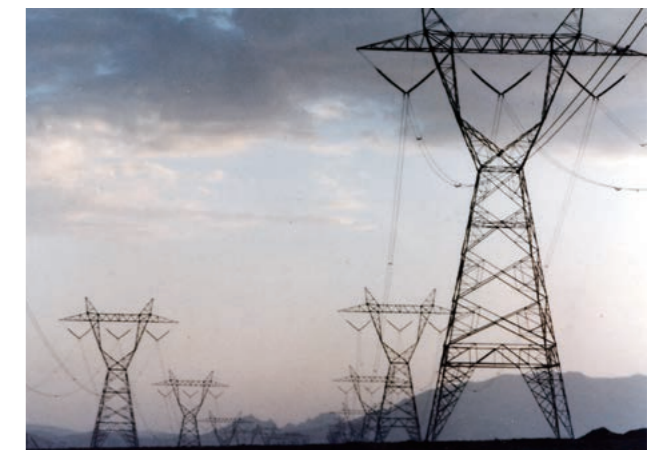
Transmission line construction in Iran
