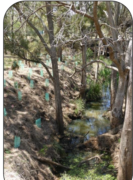
When the weeds are removed, the planting can begin.
