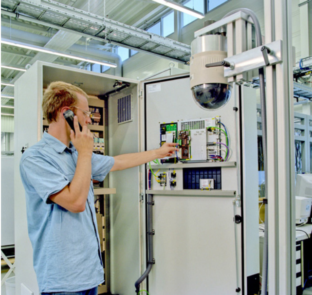
Worldwide repair service
