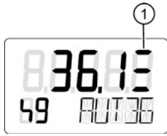
Figure 9-6 Display of a threshold 3 fault message
