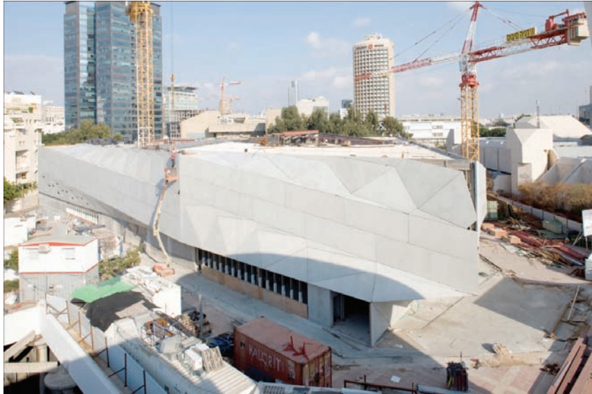
Figure 2. Overview of the construction site of the Tel Aviv Museum, showcasing the assembly of the concrete panel façade. Source: The Tel Aviv Museum of Art.
