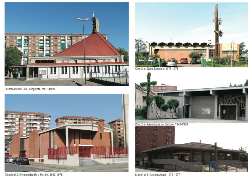
Figure 2. Parish complexes built under the episcopate of Cardinal Pellegrino, from 1965 to 1977. Source: photographs by the author
