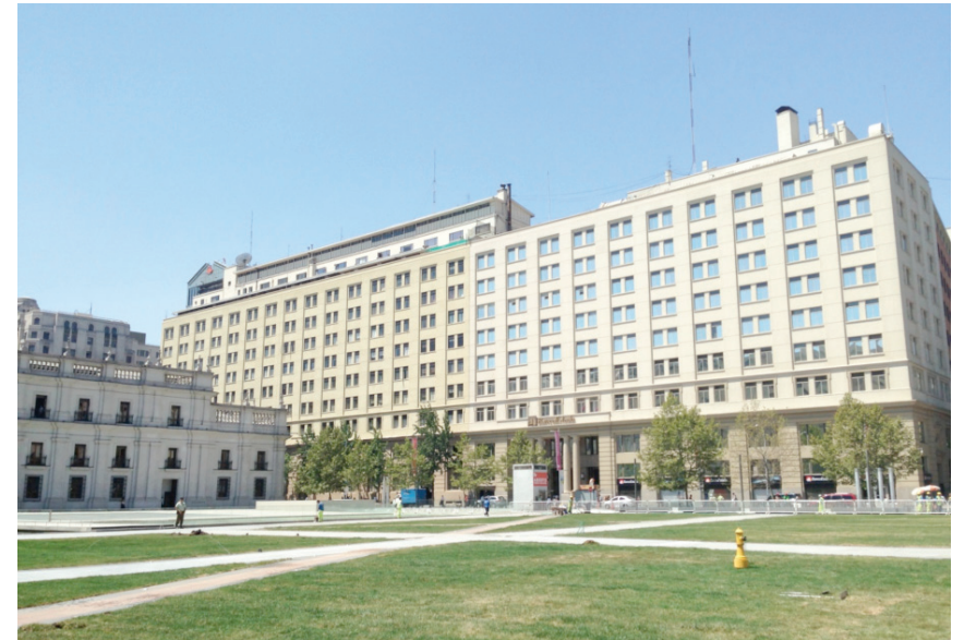
Figure 2. View of the La Moneda and the Civic District as background from Teatinos Street. Source: photograph by the author, January 2014.
