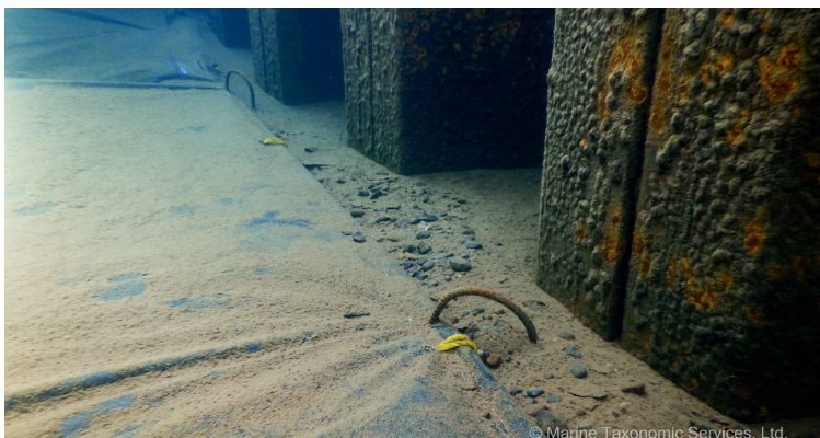
Benthic barrier installed with rebar staples at Fleur du Lac Outer Harbor
