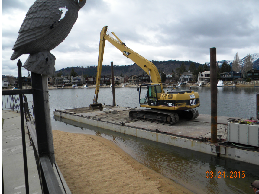
Mechanical dredging equipment at Tahoe Keys ( https://www.tkpoa.com/images/photos/projects/dredging/dredging5348.JPG )
