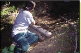
Figure 3–54—Keep stacking materials until the desired height has been reached—ideally flush with the ground level. (This photo has been digitally altered.)
