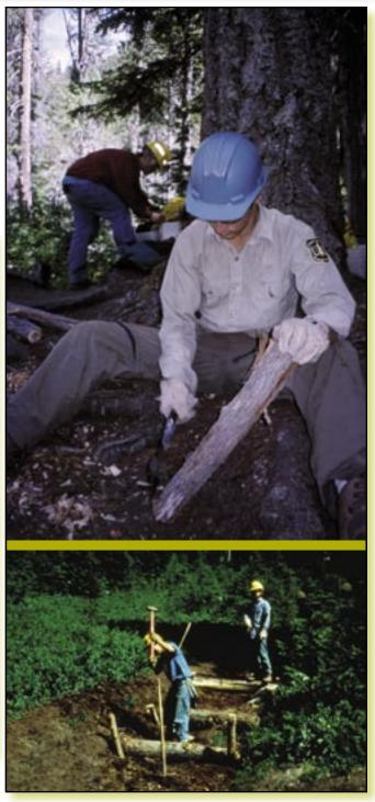
Figures 3–59a and 59b—Stout pegs are shaped with an ax or hatchet (top) and pounded into place with a sledge hammer (bottom). (This photo was digitally altered.)
