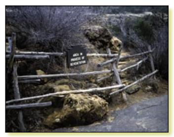
Figure 3–80—Barriers can help keep visitors from using a restoration site. This rail fence is near a road pullout at Natural Bridges National Monument, UT.
