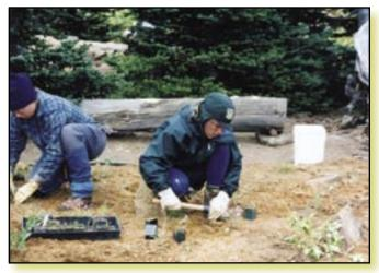
Figure 3–130—Trowels are not the tool of choice for planting. A hand-held pick hoe (shown) or plow share works well for planting smaller plants. A shovel is needed when planting larger plants.
