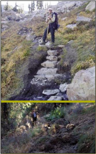
Figures 3–87a and 3–87b—Several steep, parallel trails (top) plunged down an embankment at Snow Lake in the Alpine Lakes Wilderness, WA. One trail was hardened by installing rock steps. Other trails (bottom) were closed and restored.
