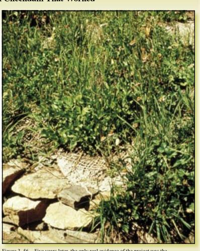
Figure 3–56—Five years later, the only real evidence of the project was the lowest checkdam.
