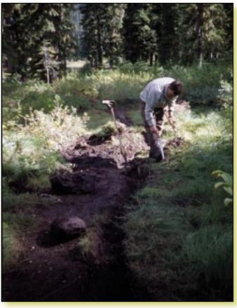
Figure 3–43—A small parallel ditch dug alongside this social trail will dry out the tread surface, reducing the likelihood that hikers will walk to the side of the trail, making it wider and wider. The salvaged plugs of plants and soil were transplanted into closed social trails nearby. The plant community may change because the water table will drop to the depth of the parallel ditch.
