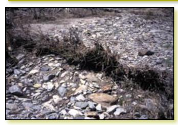
Figure 3–51—The live trench pack stabilizing this gully is one example of a living subsurface erosion control structure (Eubanks and Meadows 2002).
