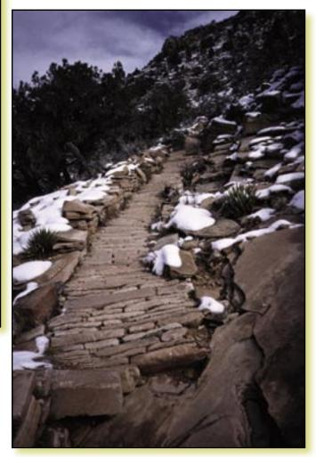
Figure 3–48—Riprap reduces surface erosion by providing a durable surface in Grand Canyon National Park, AZ.
