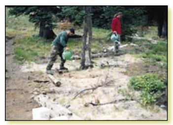
Figure 3–140a—These watering cans have the "French" handle design— a long arching handle that balances nicely and prevents back strain.
