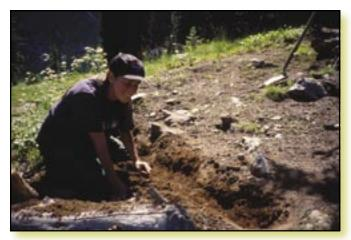
Figure 3–53a—To properly seat a siltbar or checkdam, a trench is dug about 6 inches deep across the contour or perpendicular to the gully.
