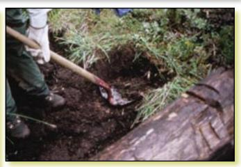
Figure 3–53b—In gullies, a keyway is excavated about 6 inches into each sidewall to pin the checkdam or siltbar material into place.
