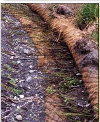
Figure 3–66—Brush layering can be used to repair an alcove where the bank has washed away (Eubanks and Meadows 2002).
