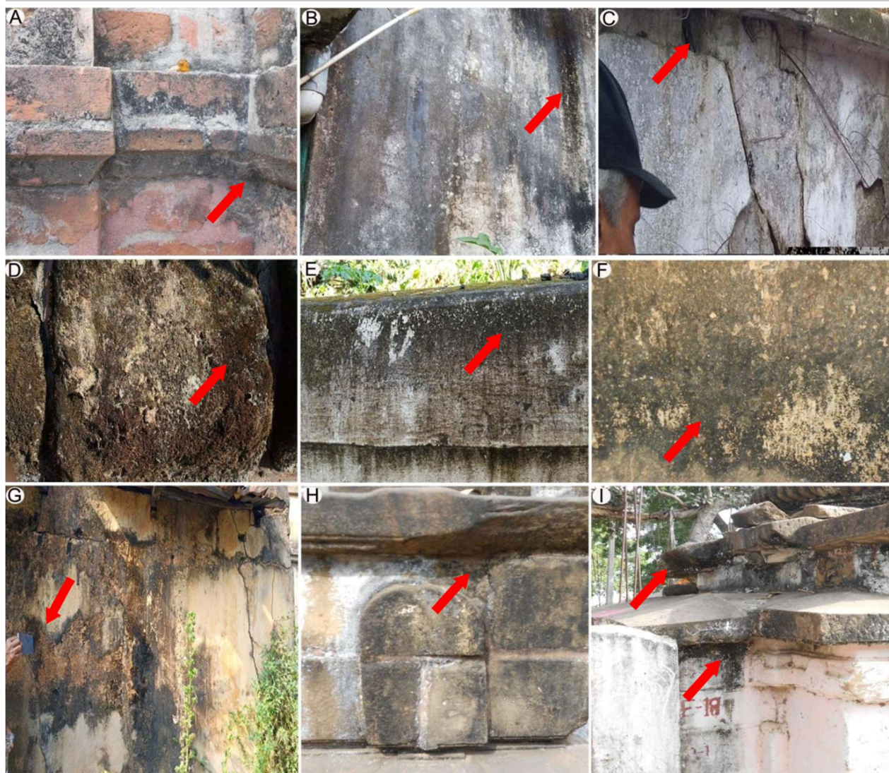
Fig 2. Photographs show the microbial biofilms on the exterior surface of monuments and building facades. A. on brick; B–C. on cement; D. on concrete; E. on limewashed; F–G. on painted surface and H–I. on stones. Arrow (↑) marked indicates to show the growth of cyanobacterial biofilms.
