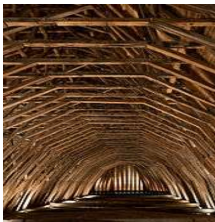
Heart of oak beams of the frame of Saint-Girons church in Monein, France
