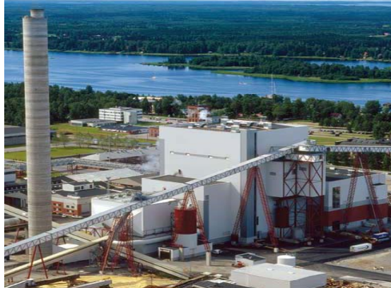
CHP paper mill
