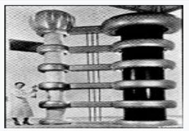
Early megavolt x-ray machine installed at Los Angeles Institute of Radiotherapy, 1938. Before linacs, high voltage x-ray tubes *(left column)* powered by million volt transformers *(right column)* were used to produce penetrating xrays
