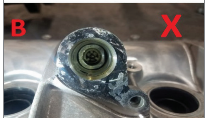
A. Clean bore B. End of solenoid stuck in the bore
