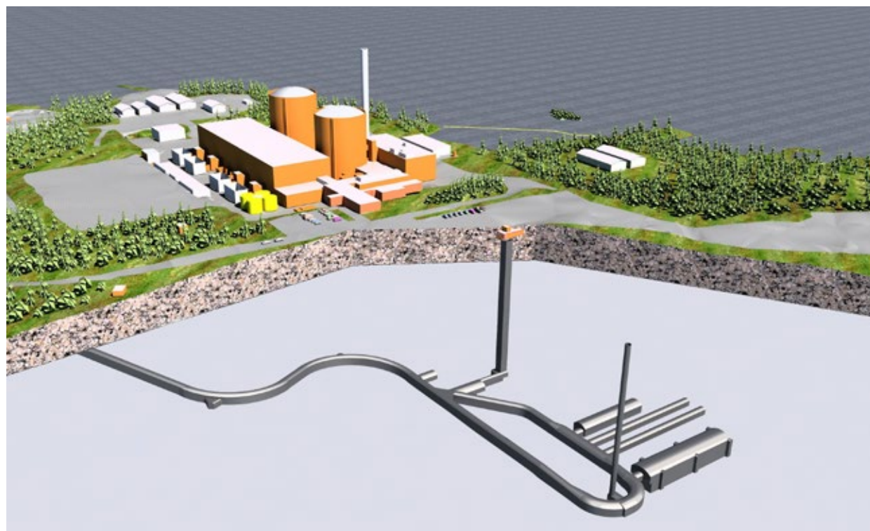
Figure 3-4. The final disposal facility for low- and intermediate-level waste in Loviisa. Layout: Timo Kirkkomäki, Fortum.
