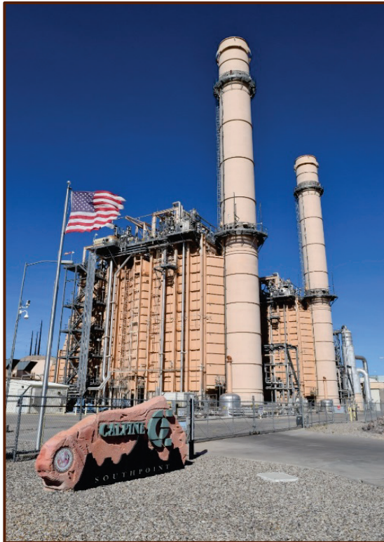
The Southpoint natural gas-fired electric generating plant at the extreme SE corner of the Fort Mojave Indian Reservation.
