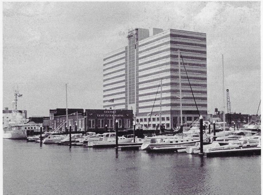
Closeup view of Newport Marina today as construction continues in the background.
