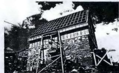
◀ Construction of solar-electric plants for remote buildings
