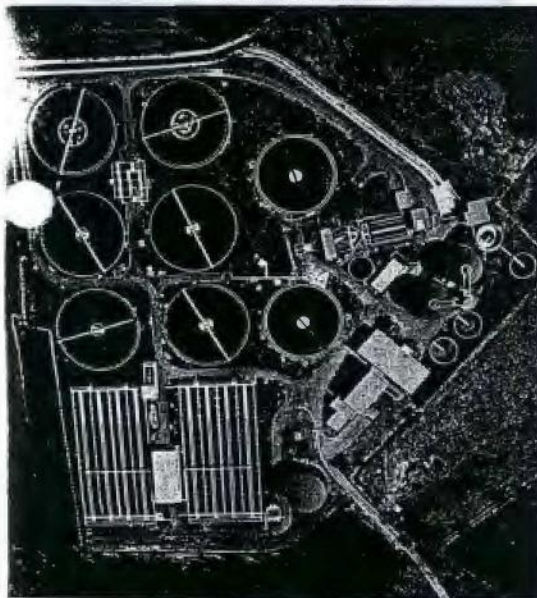
Dornbirn Wastewater Treatment Plant, Austria 1983. Population equivalent: 280,000. Mechanical and chemical treatment. ▼
