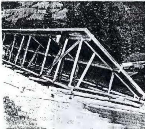
▼ Structure of aluminium components for collector installation ▲
