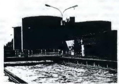
▲ ARA waste water clarification plant in Feldkirch/Austria
