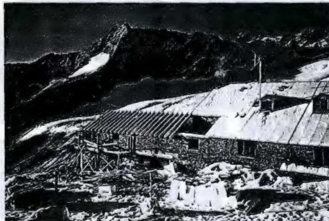
▲ Construction of dry toilets in Kaunergrat Hut
