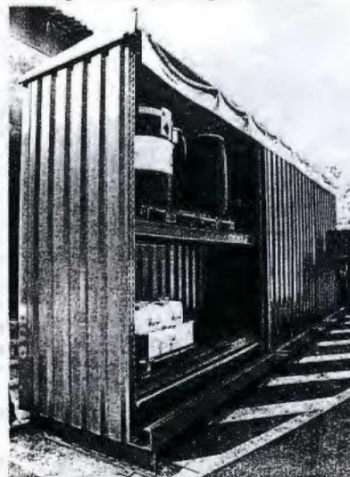
Storage of water-polluting materials
