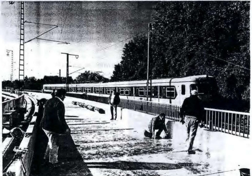
▼ Laying Sylomer® sub-ballast mats on a high-speed railway bridge
