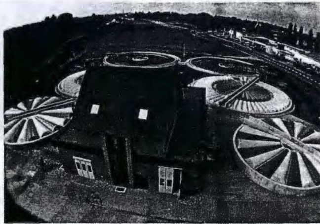
The Eberstadt sewage works with Phostrip pool ▲
