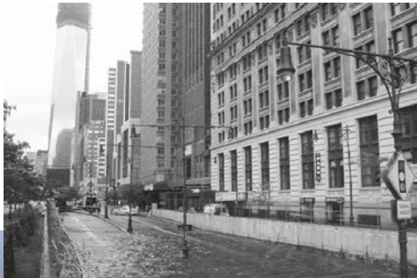
Flooding of the Brooklyn Battery Tunnel, looking northward, toward the unfinished Freedom Tower, 2012 (Photo credit: ARCADIS)
