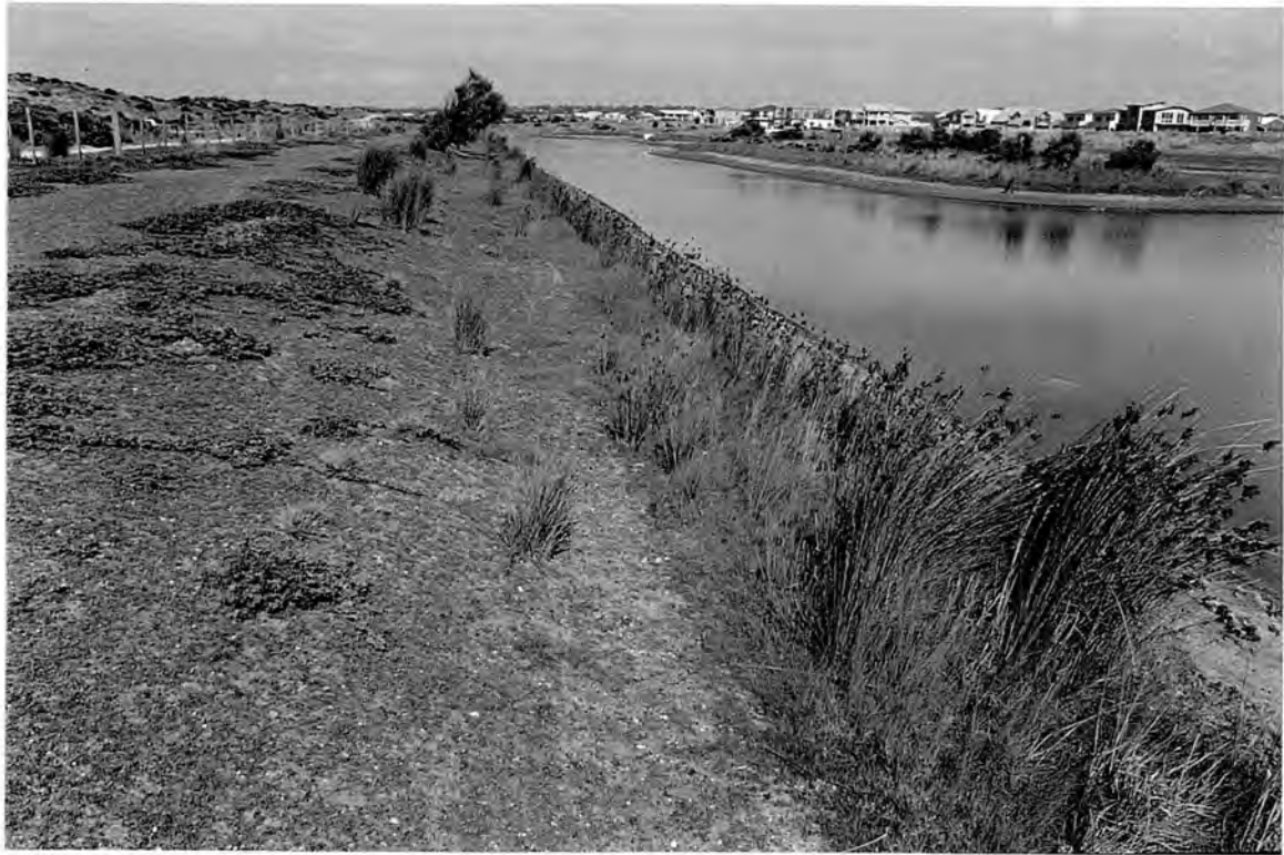
Plate 15. The constructed wetland associated with the current residential development. A near-total absence of wetland vegetation and intense rabbit grazing are evident.
