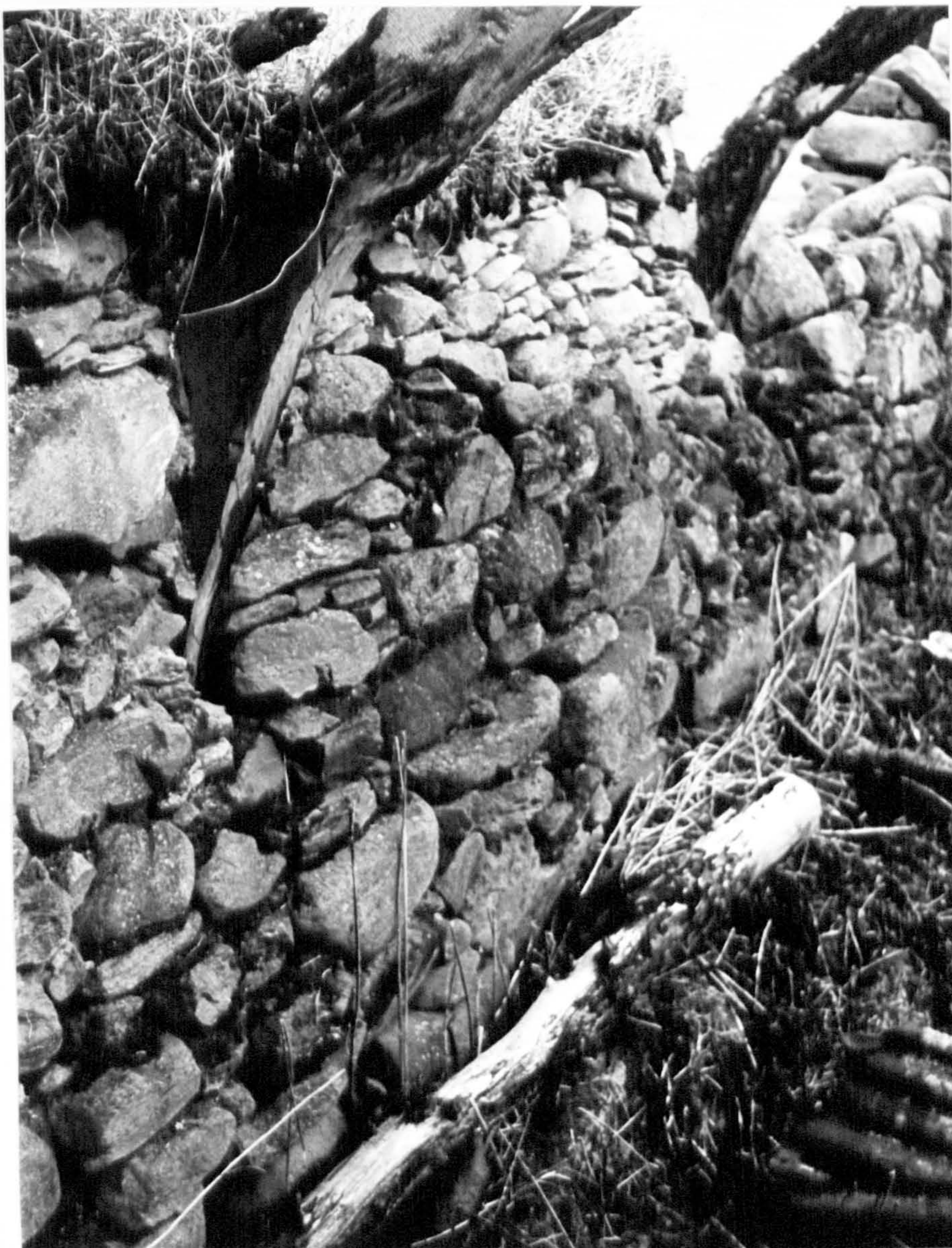
Plate 29. Feet of crucks in wall slots, west and central crucks, North wall of Section A 1 , Building A in Cluster B on Cuiltrannich, 1966 (Figure 31).
