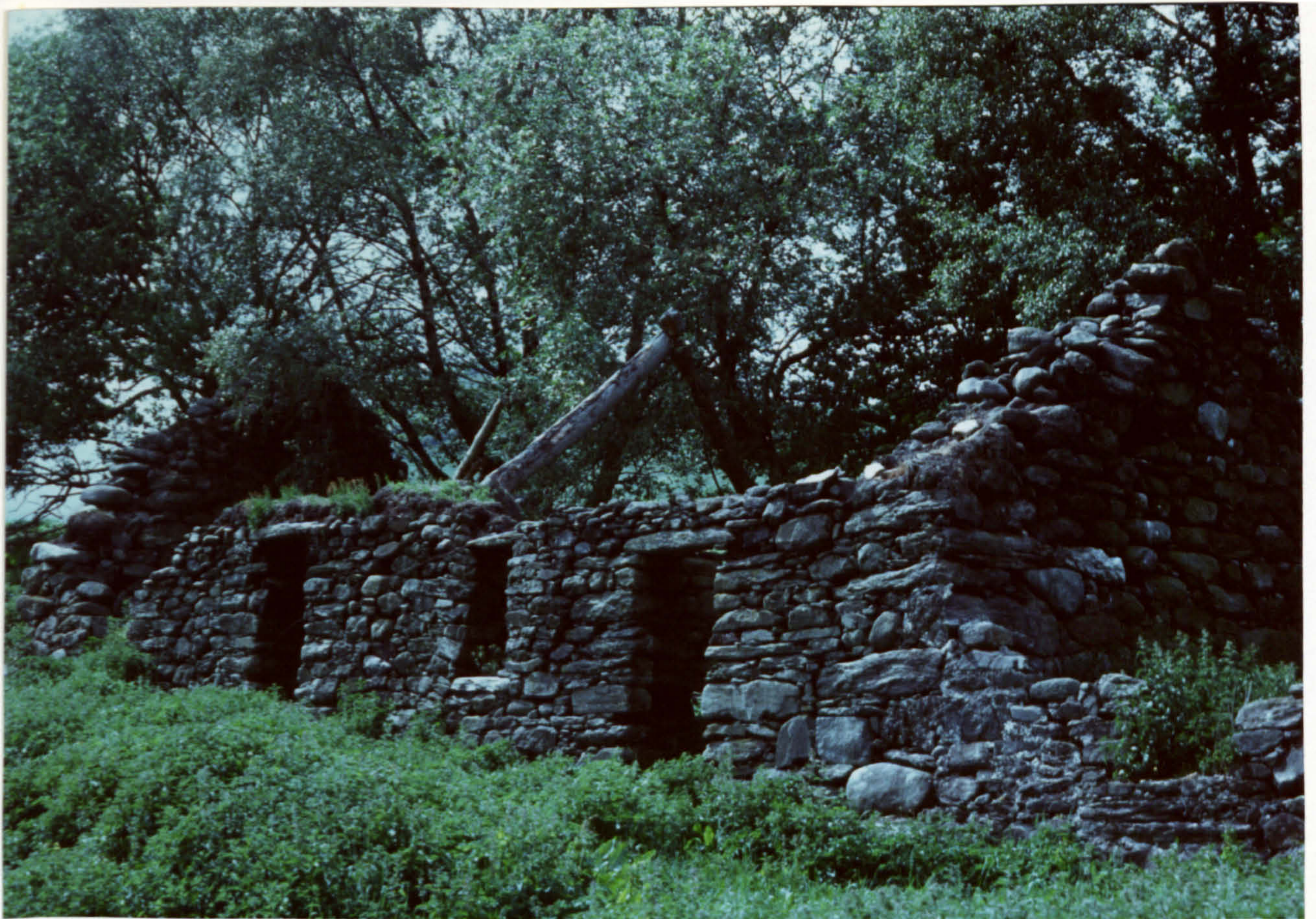
Plate 23. Building A in Cluster B on Cuiltrannich in 1978. Only one cruck couple still remains in position, the roof is entirely gone and the walls of section A 2 (Figure 31) have almost completely collapsed.
