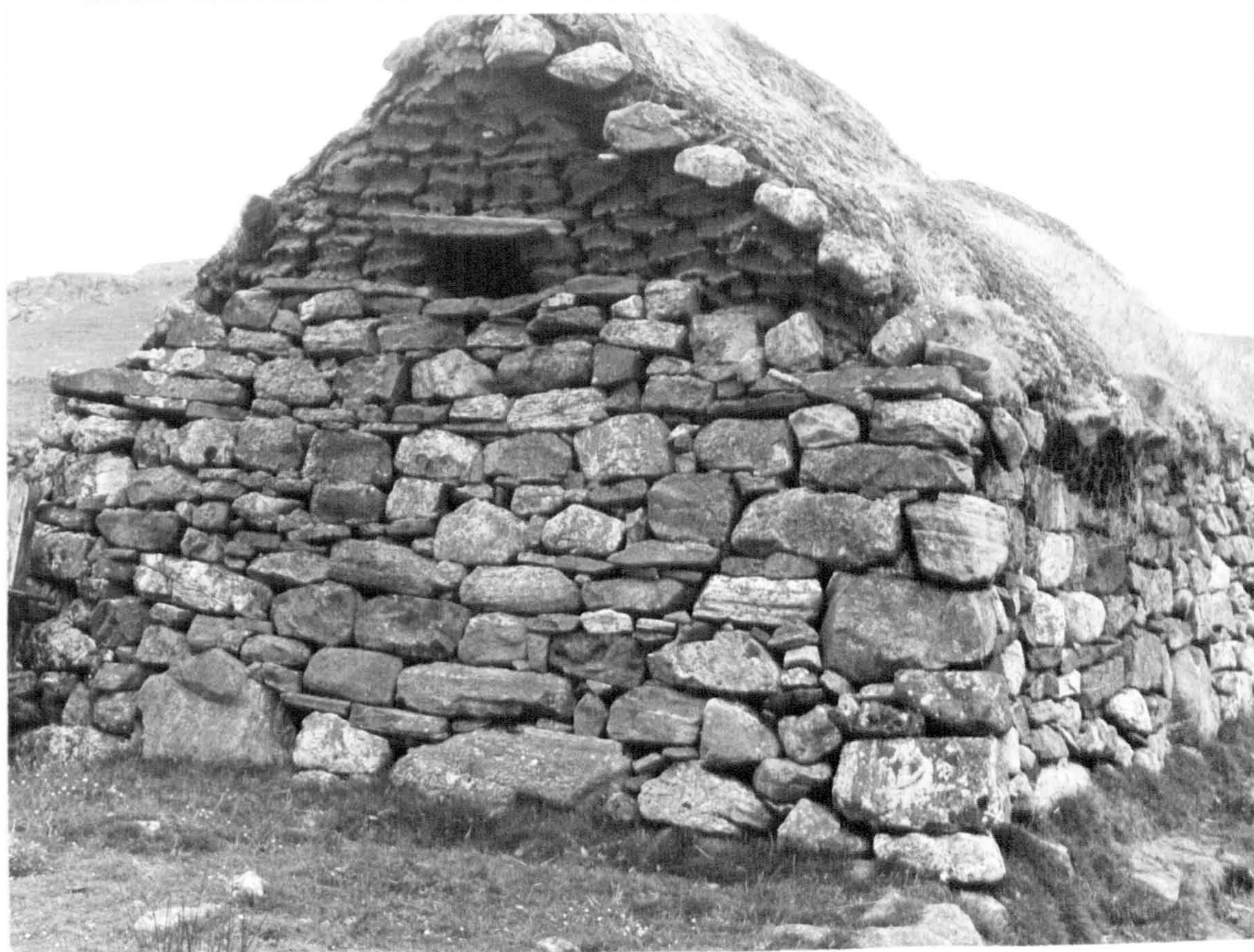
Plate 60. Old building on Clashnessie, now used as outhouse. Upper gable of turf.
