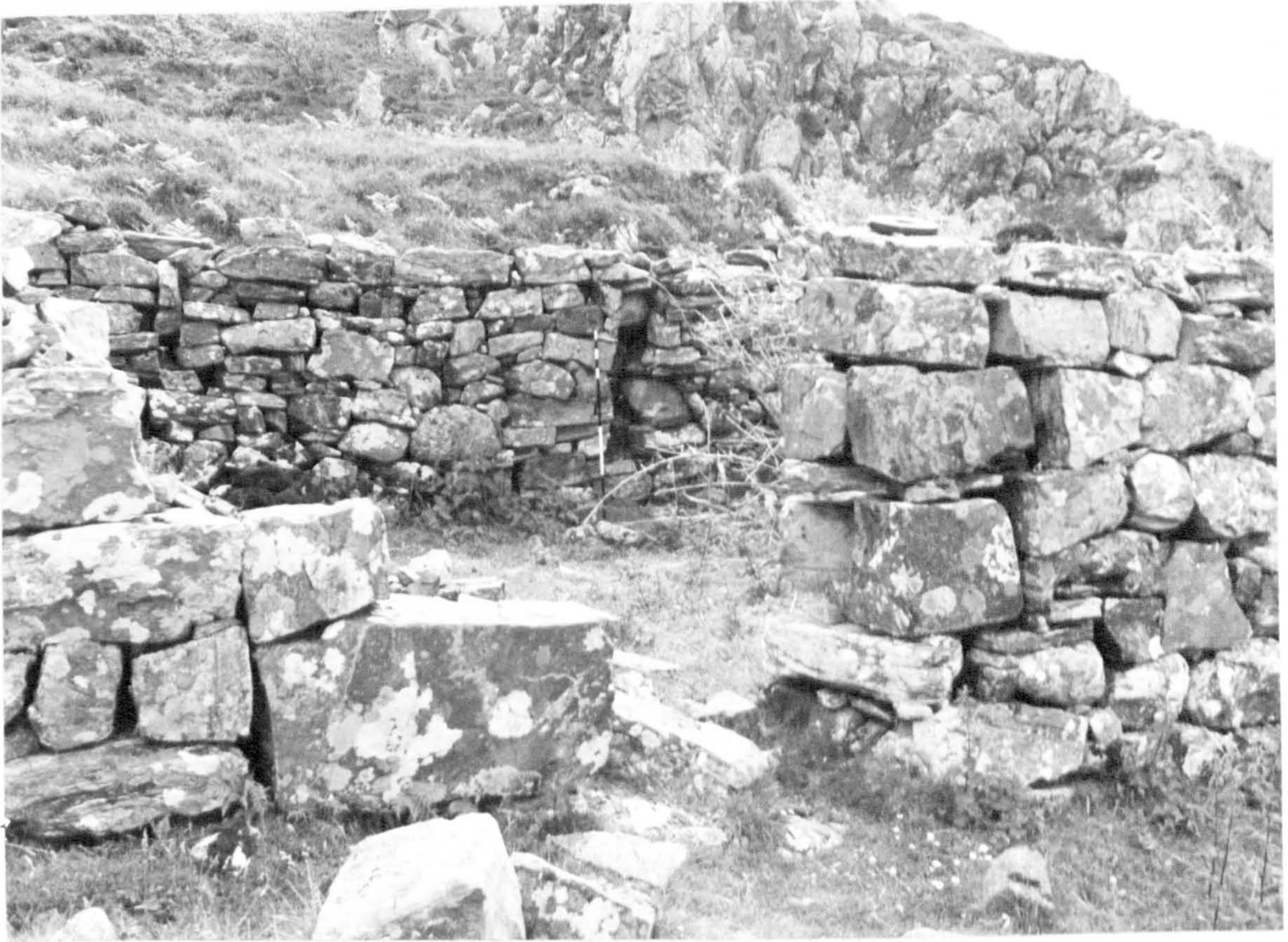
Plate 82. Interior of Building E, Glananter sheeling, showing single cruck slot in SE wall.
