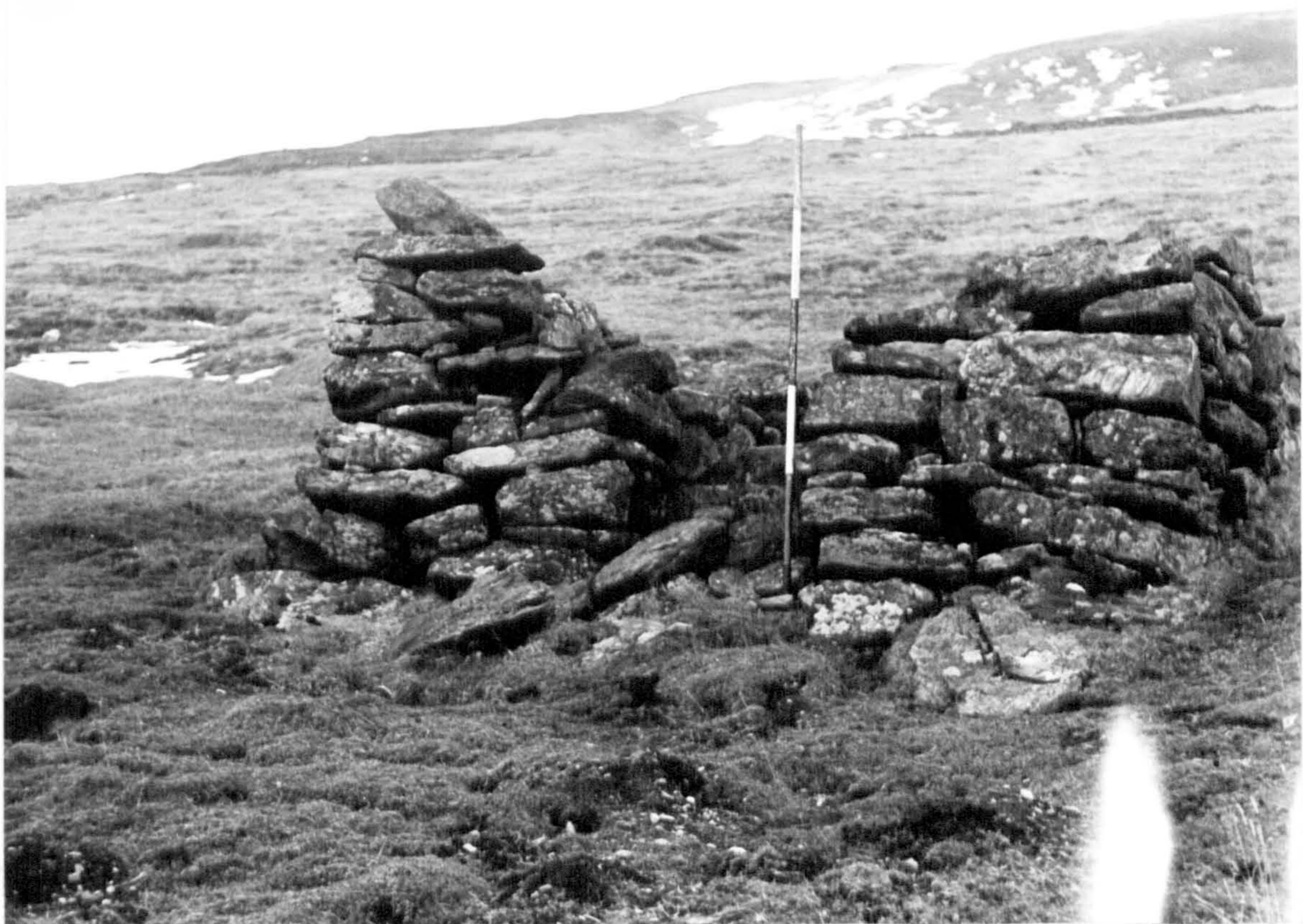
Plate 52. Structure Y, possible shieling bothy (Figure 48), modern head dyke in background. Ranging pole in feet.
