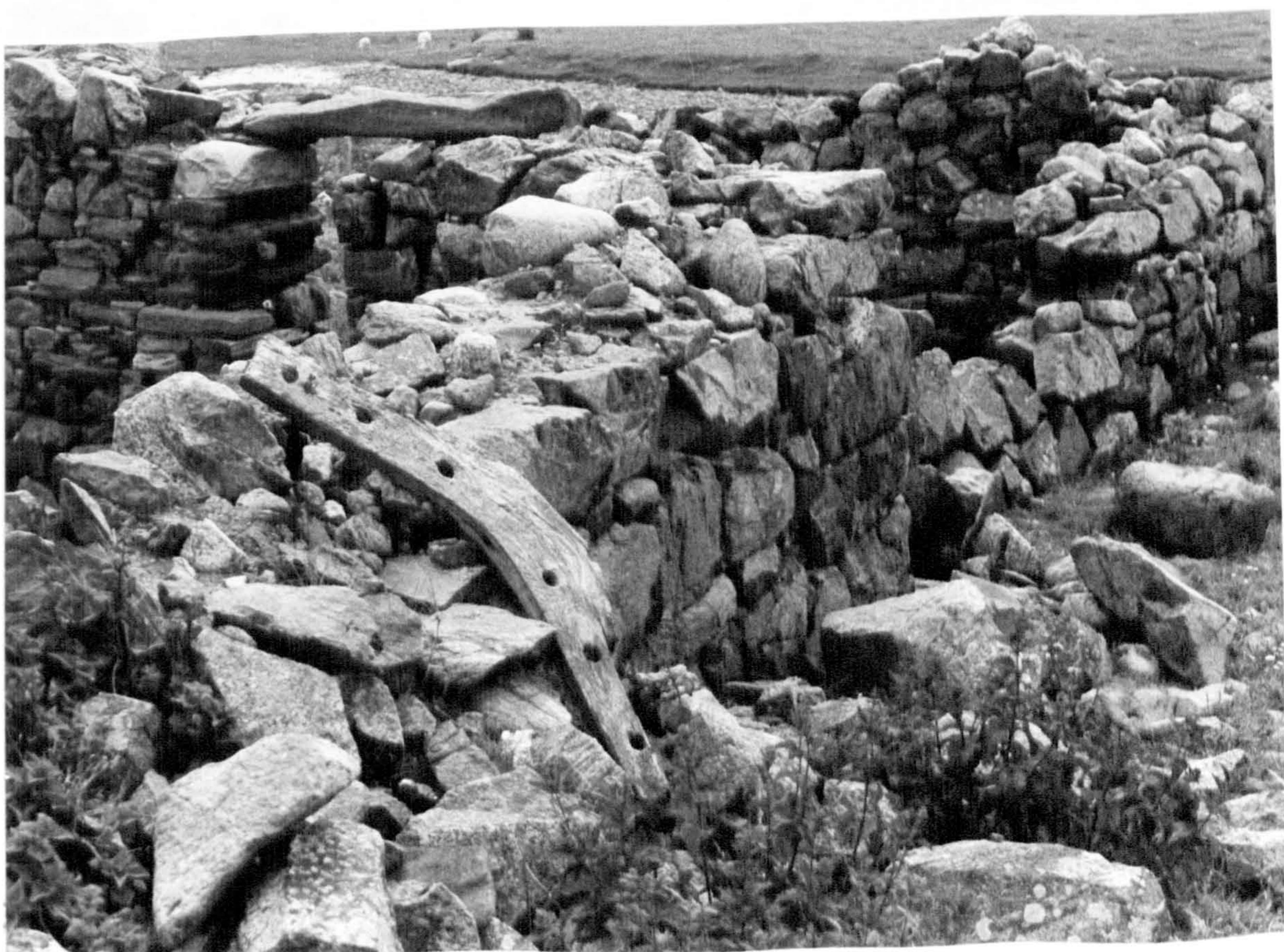
Plate 79. Remains of cruck with pinning holes outside wall of building at X on Auchmelvich (Figures 67 and 68).
