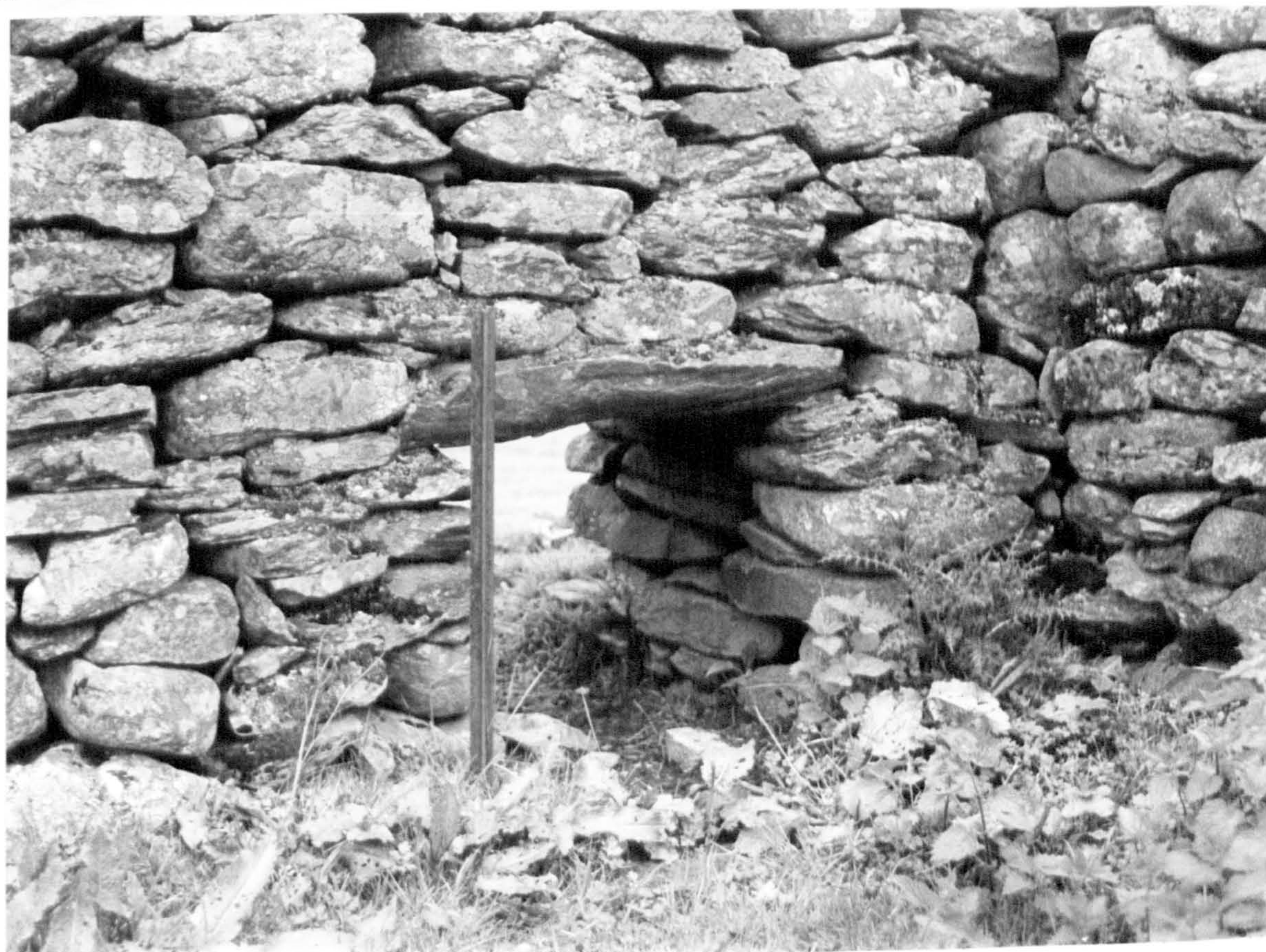
Plate 41. Interior of Building B in Cluster A on Newton Farm, showing possible winnowing-hole or toll fhasgnaidh .
