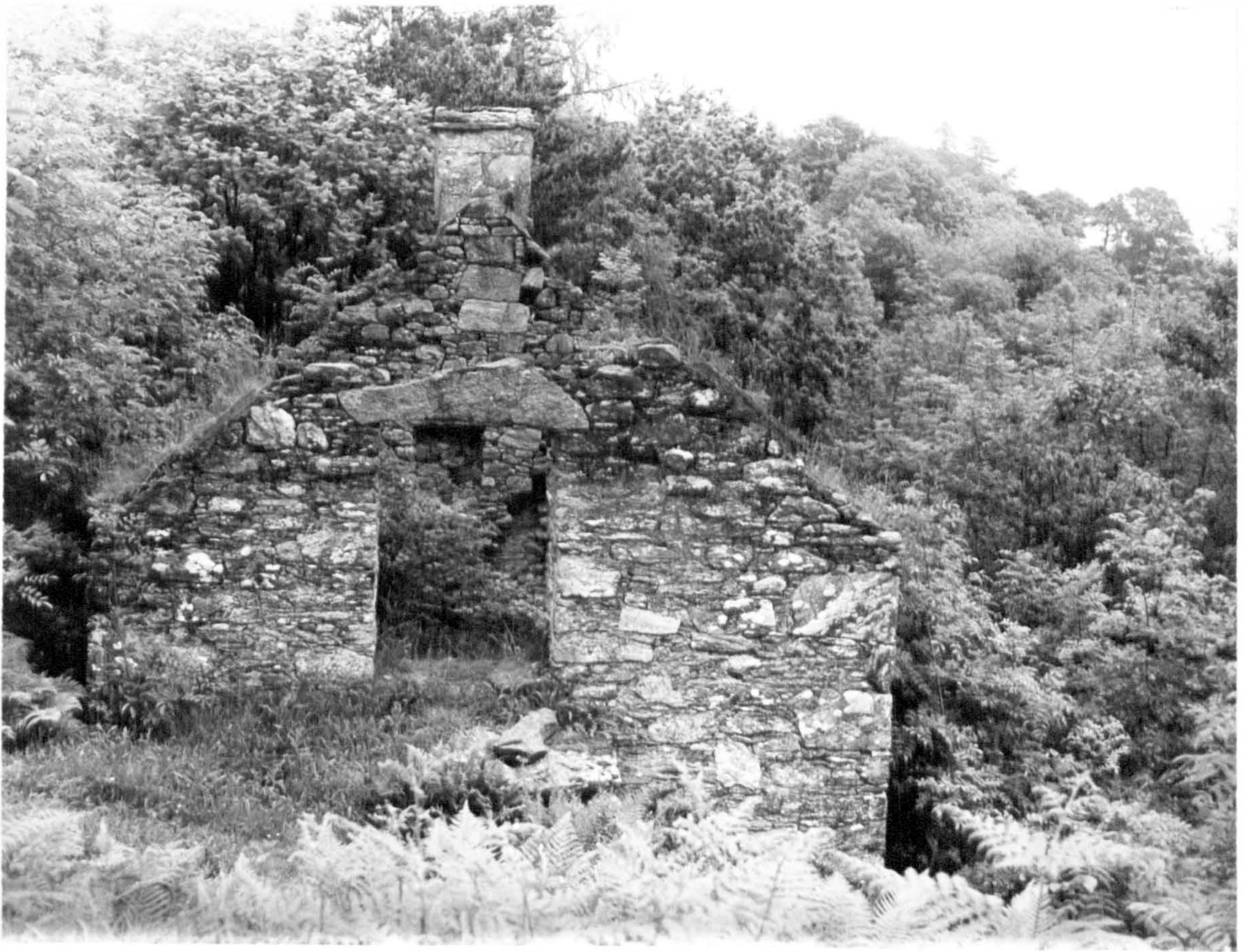
Plate 7. Building C in the northern part of Cluster A on Blarliargan.
