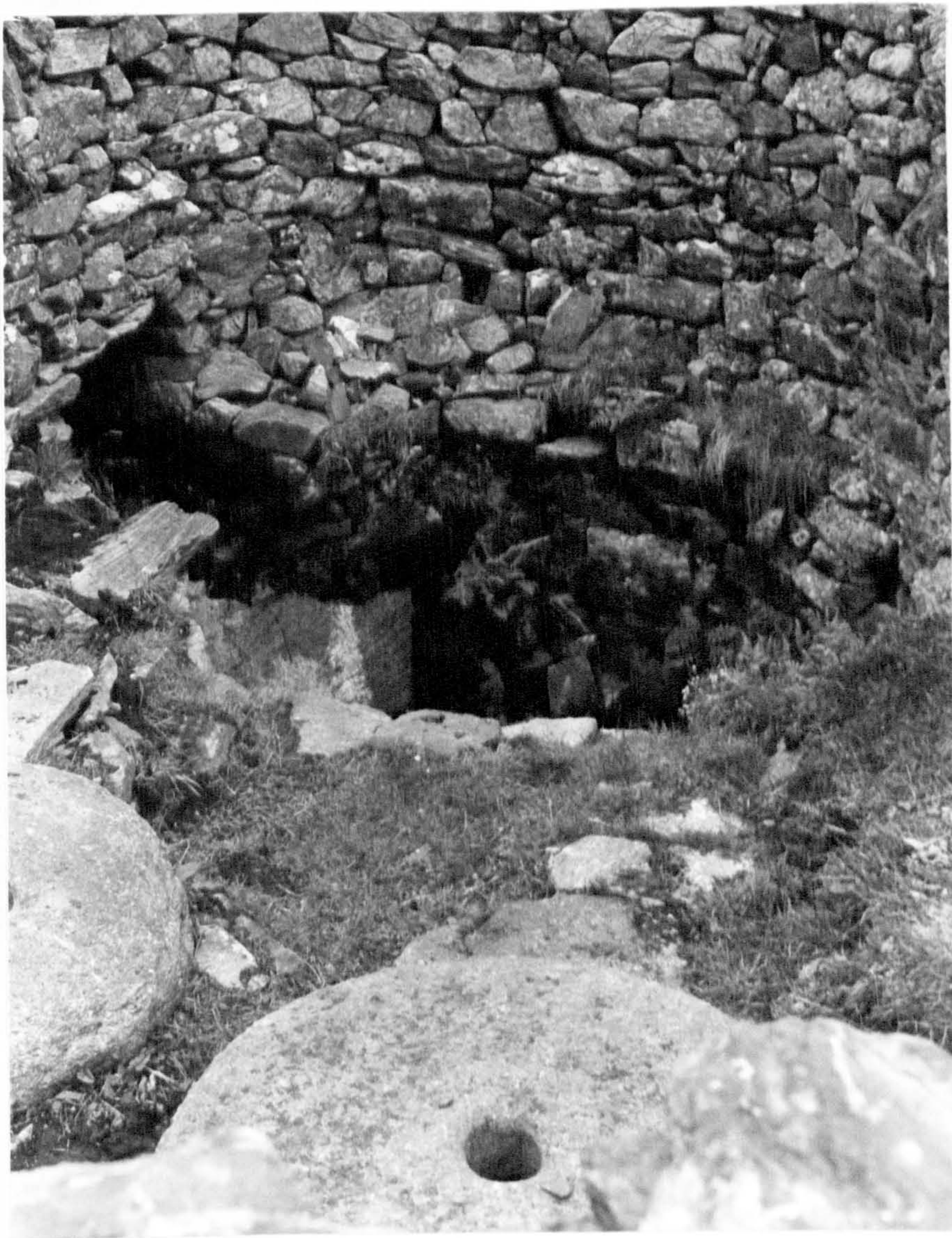
Plate 97. Basin for horizontal mill-paddle, interior of ruined mill on Alltanabradhan Burn.
