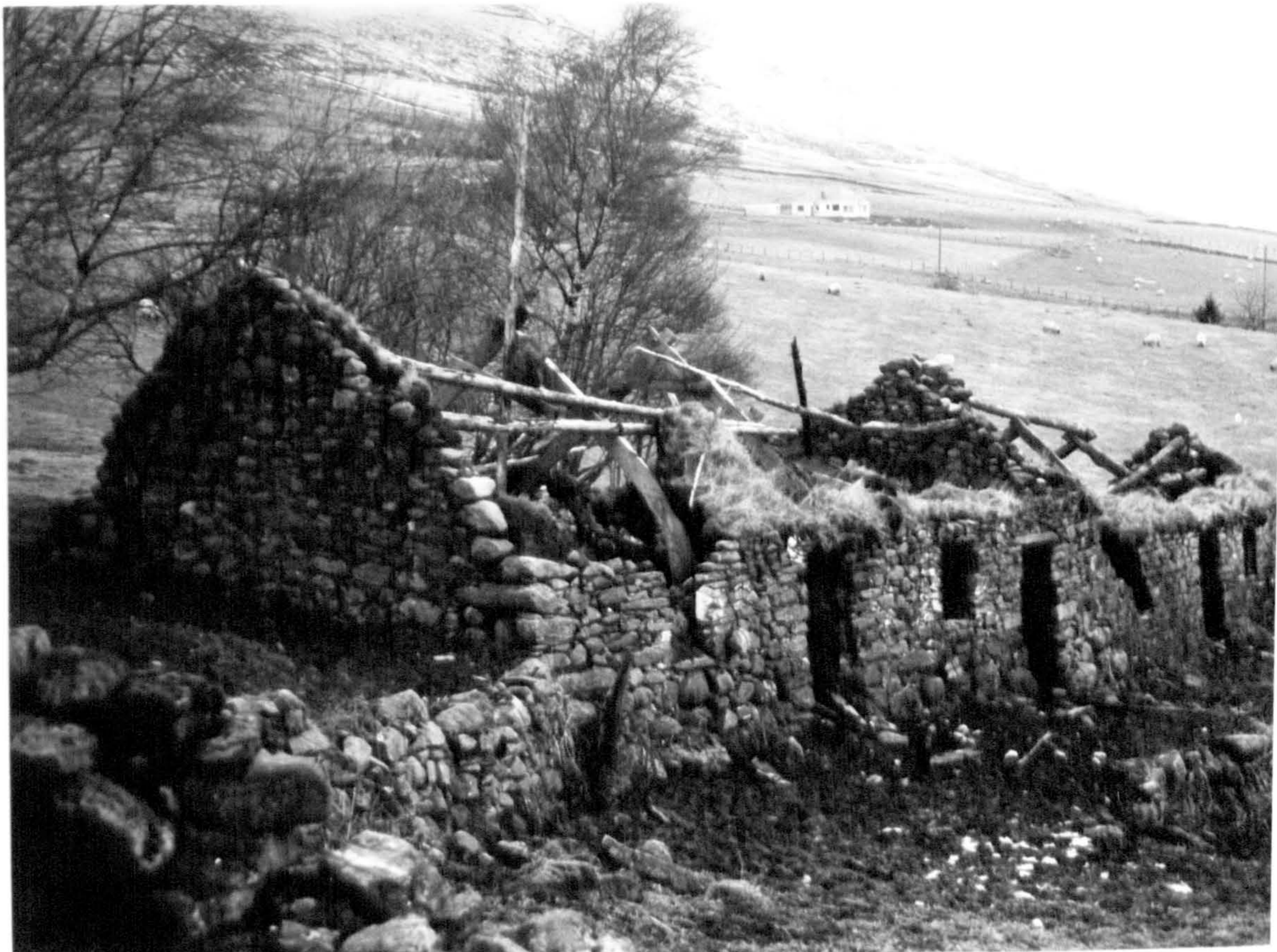
Plate 22. Building A in Cluster B, Cuiltirannich in 1966. The roof covering, now almost completely disappeared, had probably been turf under straw thatch (sgrathan). The upper crucks still carry remnants of purlins and the roof tree.
