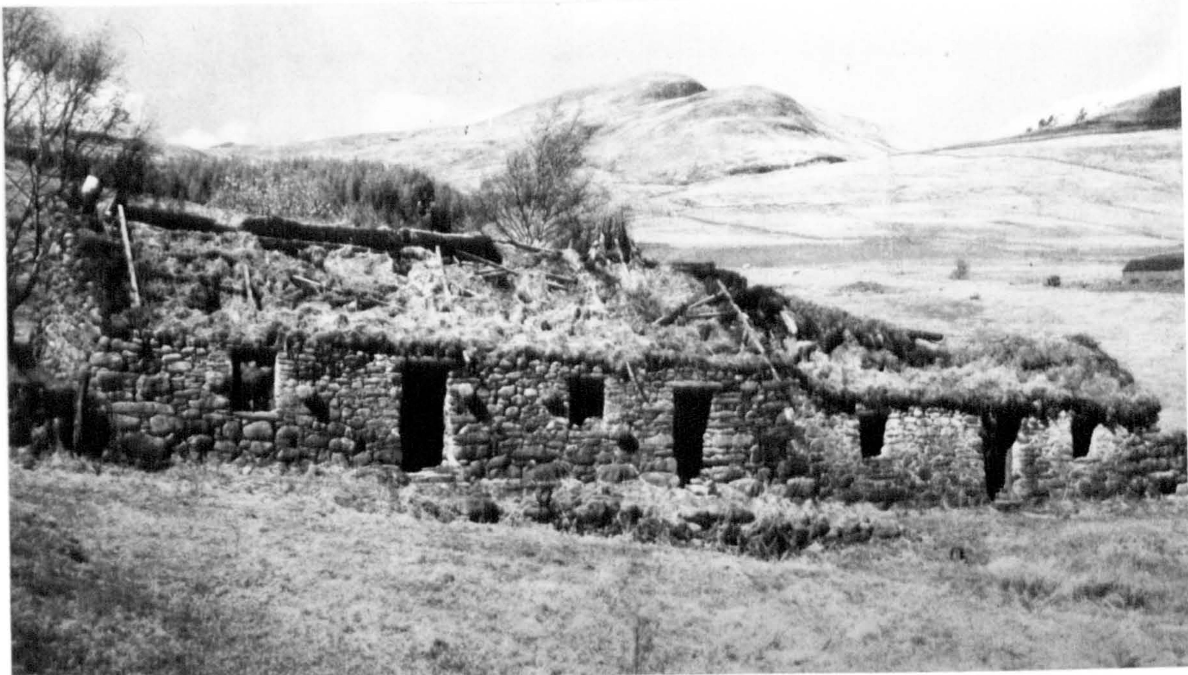
Plate 21. Building A in Cluster B on Cuiltirannich (Figure 31) in c. late 1950's. The doors and window frames have gone, the roof covering has deteriorated and the rafters and crucks are showing through, but some of the of the suspended stones which secured the earlier thatch have survived in situ. (Dunbar, 1966).
