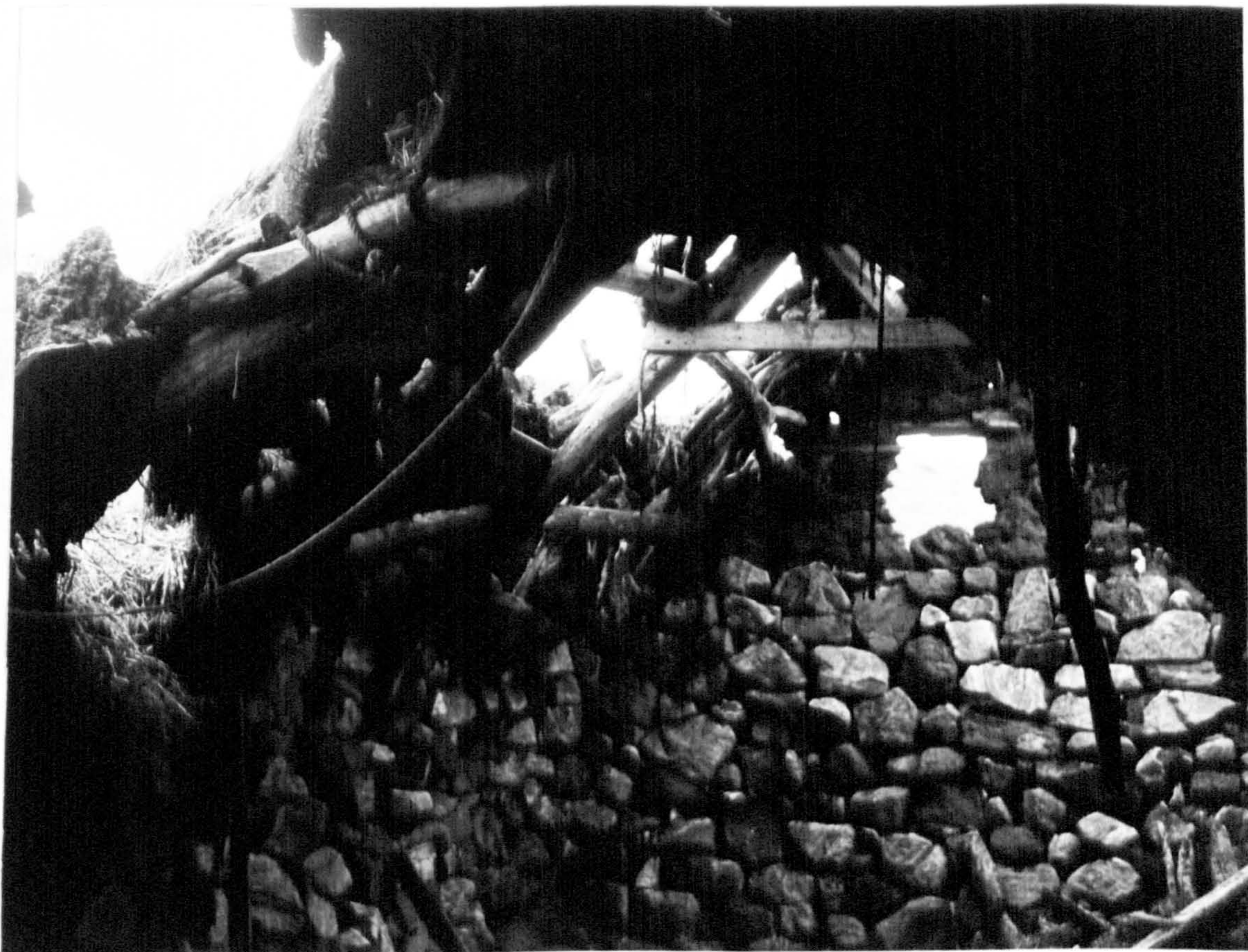
Plate 59. Interior of Building A on Clashnessie (Plate 58). The crucks are in a somewhat dilapidated condition, but at least one collar beam is still in place. Turf upper gable in background.
