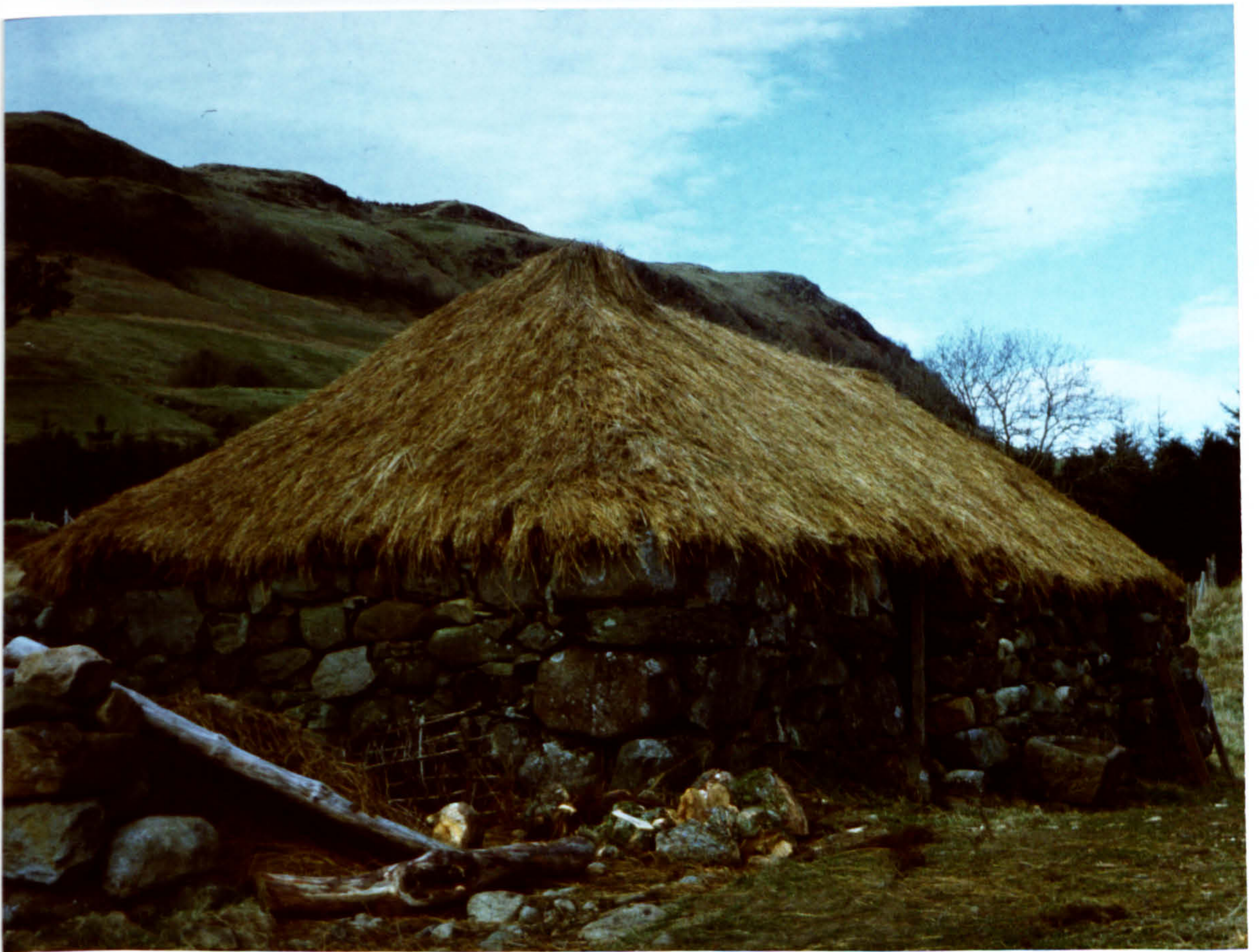
Plate 106. Building G at Auchindrain, reconstructed with hipped roof, crucks and central hearth. Thatched with straw on heather.
