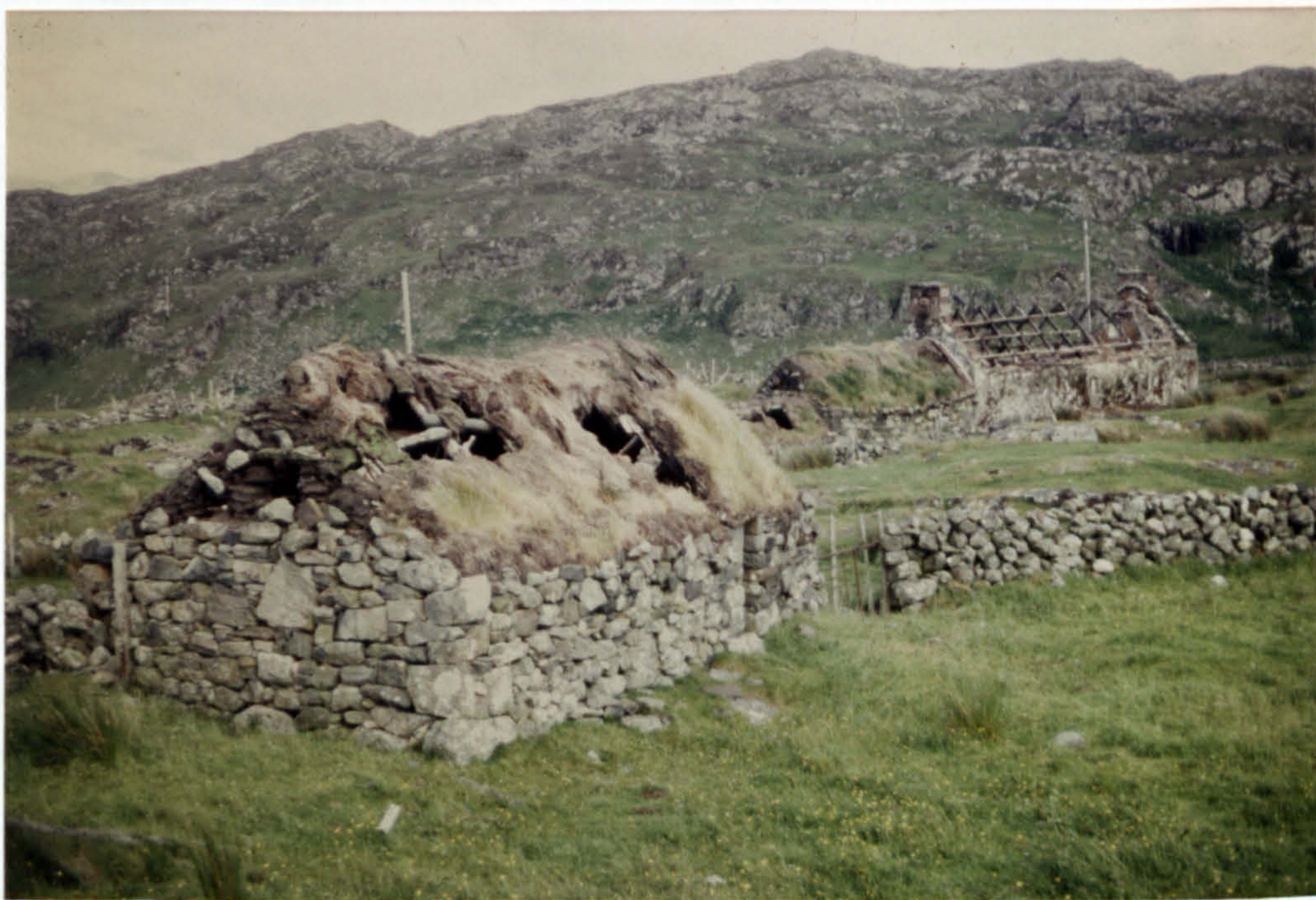
Plate 58. Building A on Clashnessie (Figure 60). An old style of construction with the upper part of the gable ends and the roof made of turf. The roof is supported on crucks (see Plate 59) unlike the later unroofed house in the background which has normal rafters resting on the wall heads.
