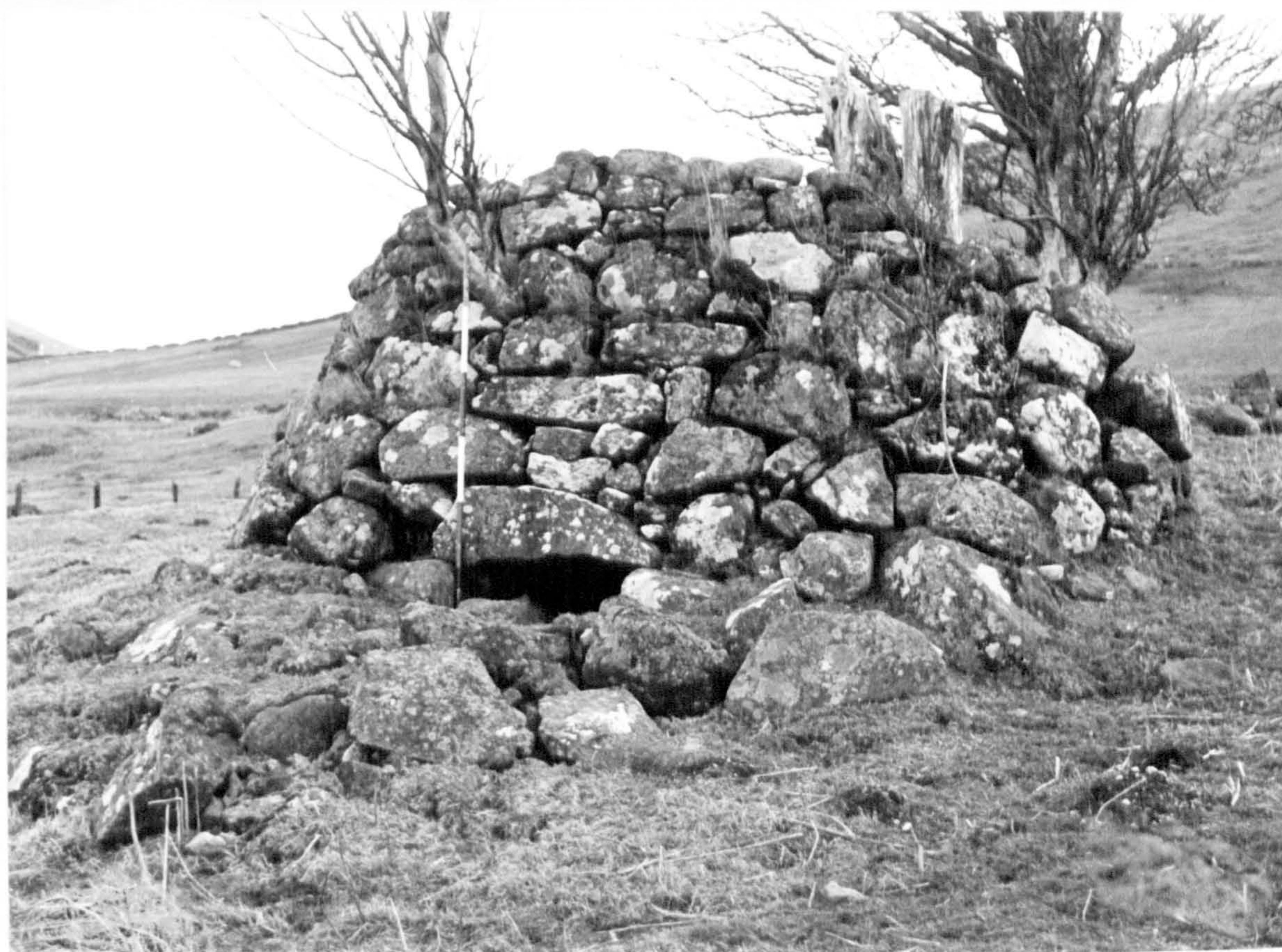
Plate 49. NW end of Building D on Craig Farm (Figure 46). Long house 64 x 17½ feet at NW end which has corn-drying kiln.. Ranging pole in feet.
