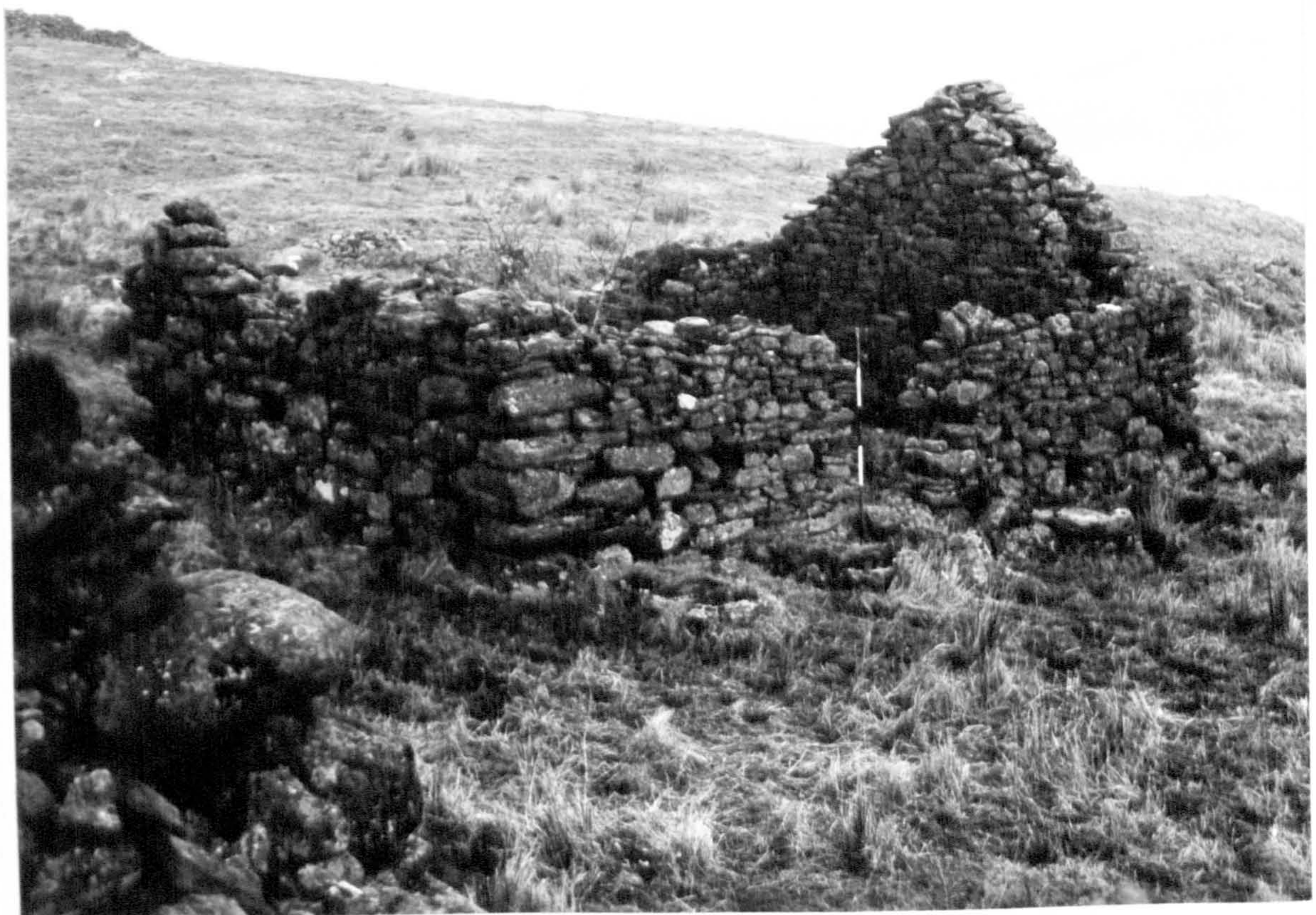
Plate 16. Building B, possible barn, on Marrag Dow cluster, Wester Carawhin (Figure 27).
