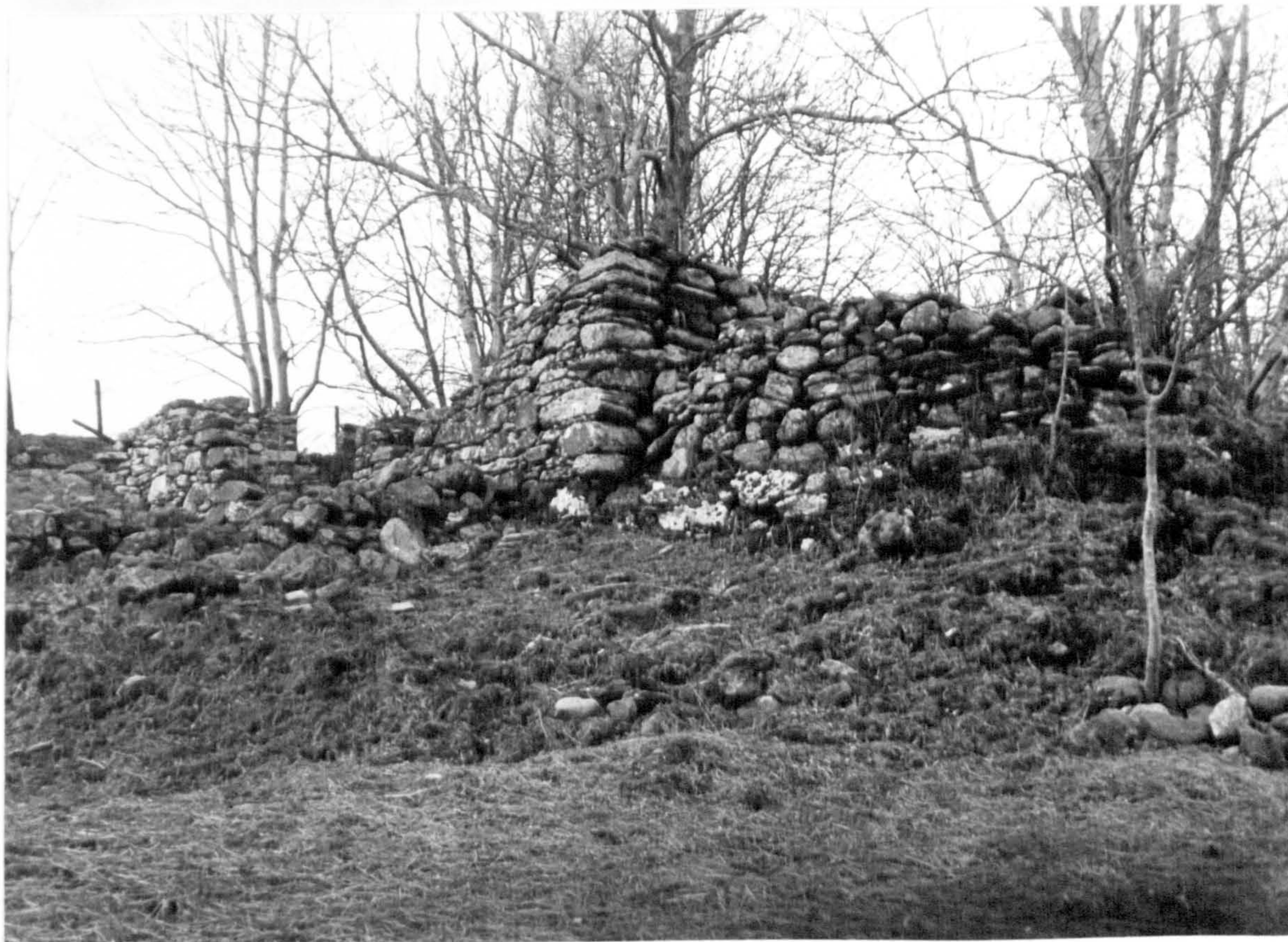
Plate 36. Lawers Mill, with remains of corn-drying kiln attached to NE end
