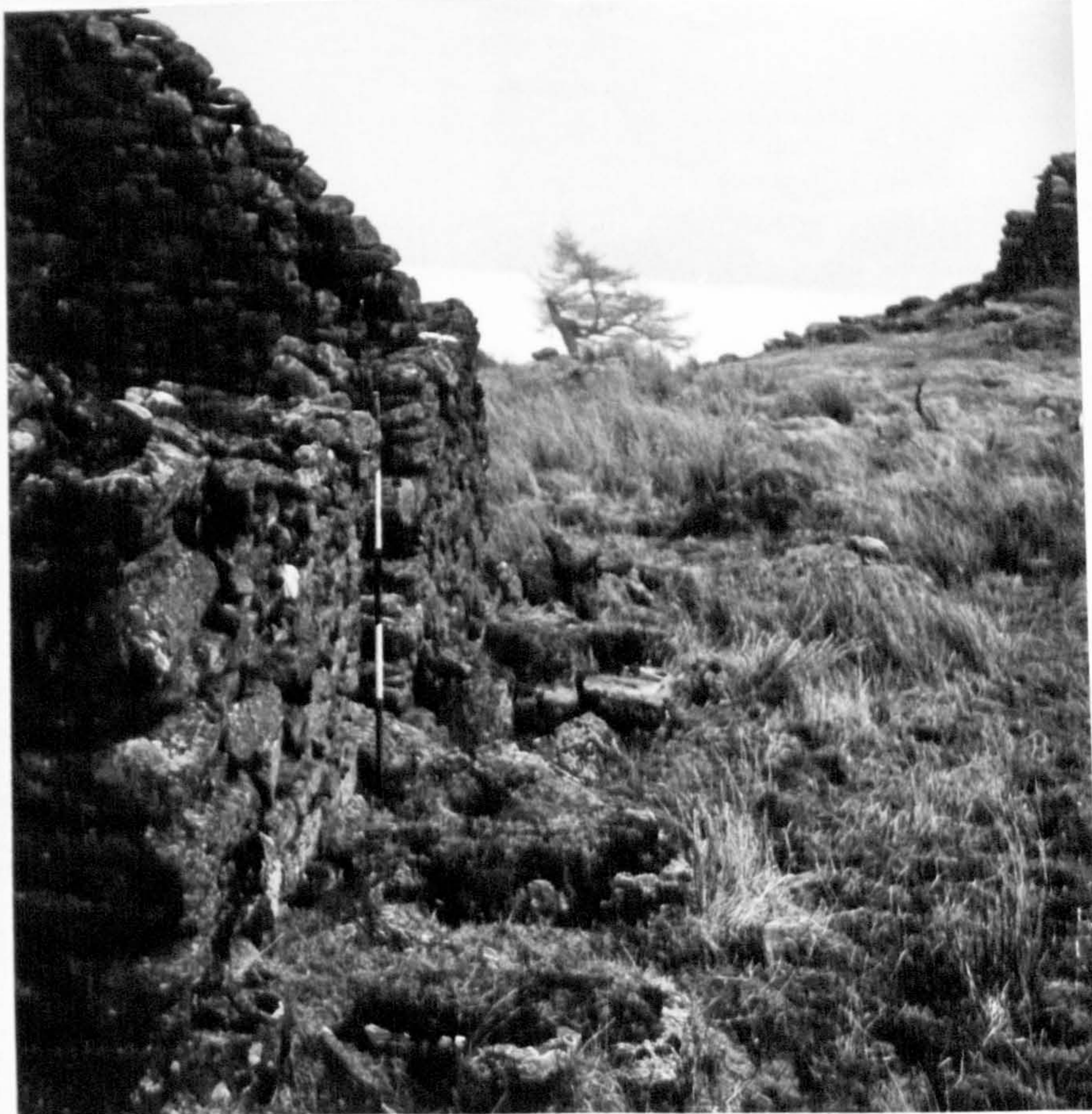
Plate 17. Building B in Marragow cluster, Wester Carawhin, showing 5 dry-stone 'piers' along western wall (Figure 27). Ranging pole in feet.
