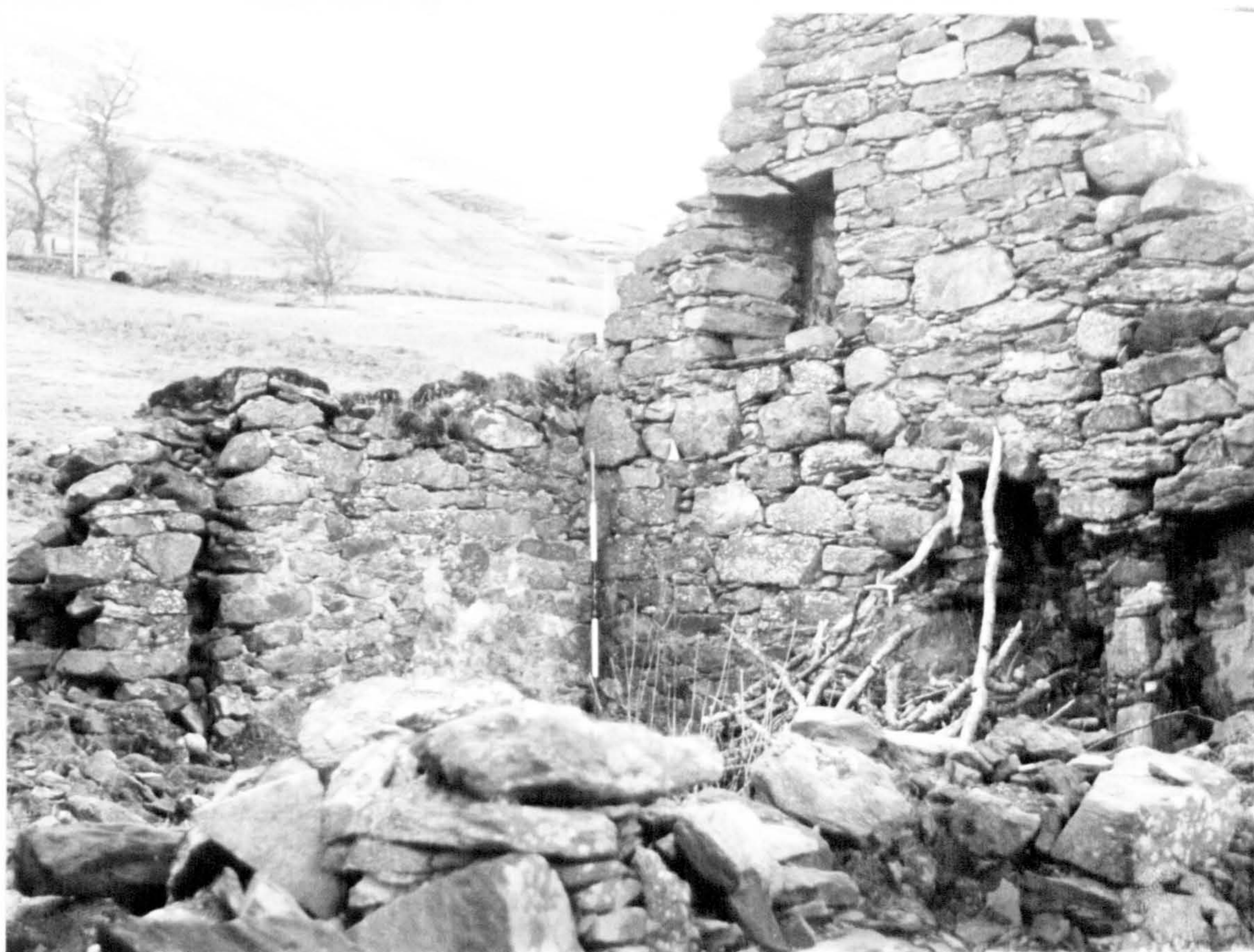
Plate 47. Interior of Building A in Cluster B on Craig Farm. Loft window and fireplace in SW gable end. Cruck slot in mortared wall. Ranging pole in feet.
