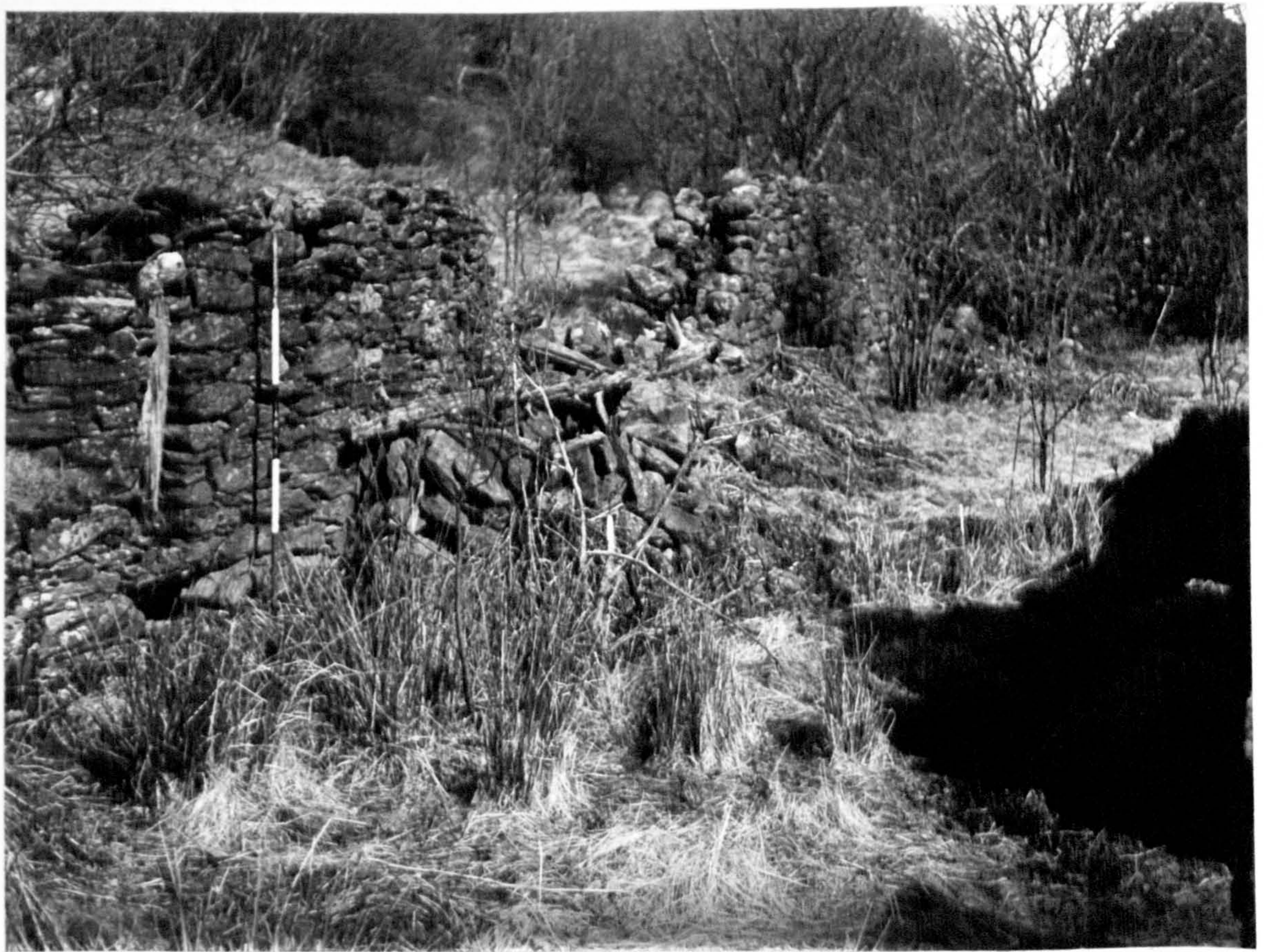
Plate 11. Remains of Building A in Cluster B on Wester Kuilturie. The ranging rod (in feet) stands beside the surviving lower part of a cruck couple.
