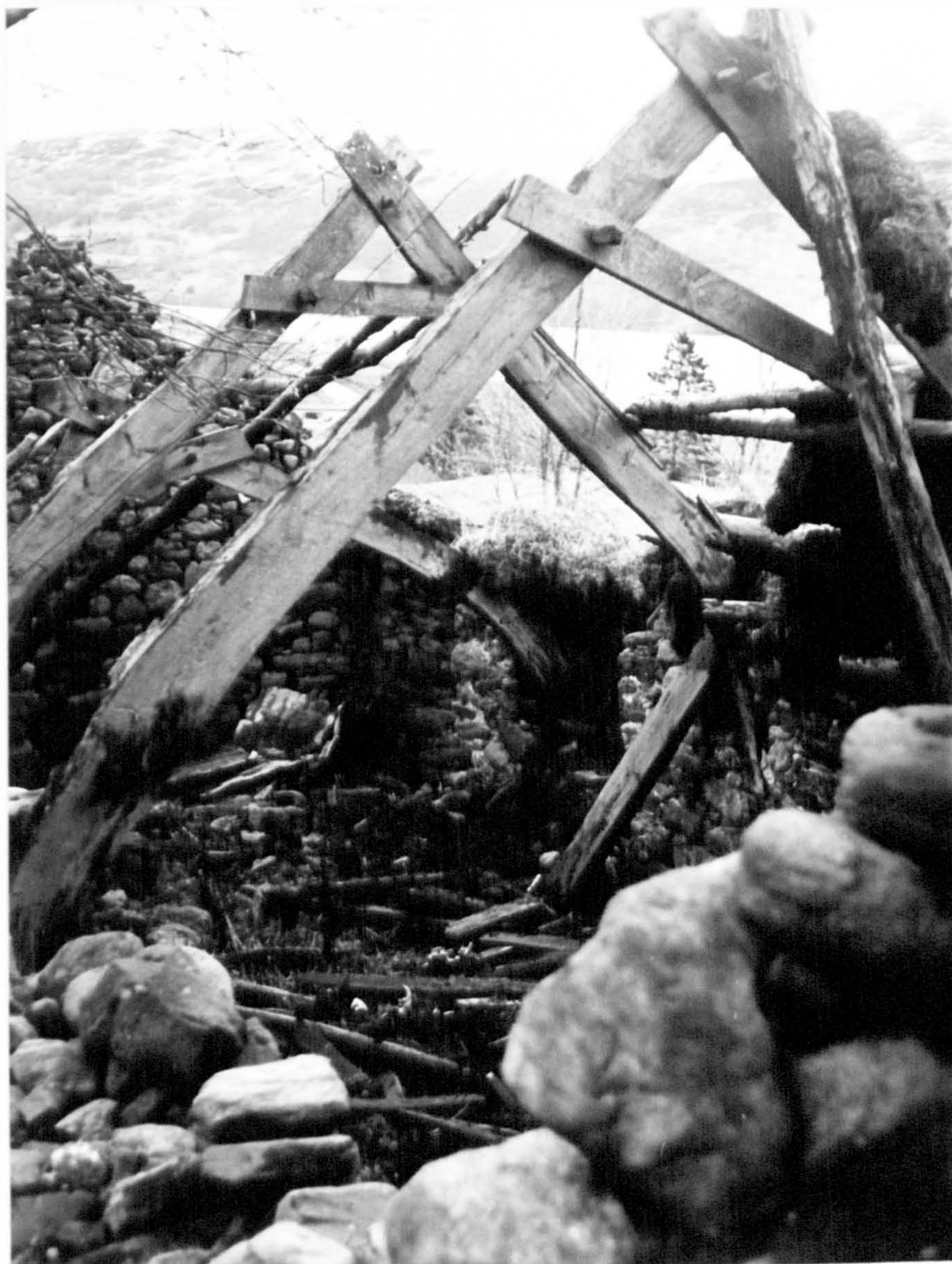
Plate 25. Interior of Building A in Cluster B on Cuiltrannich in 1966, looking east (Section A 1 in Figure 31). Three cruck couples are still in position although the rearmost has slumped from one of its wall slots. The collar beams or ties and crossed couples are secured with wooden pegs.
