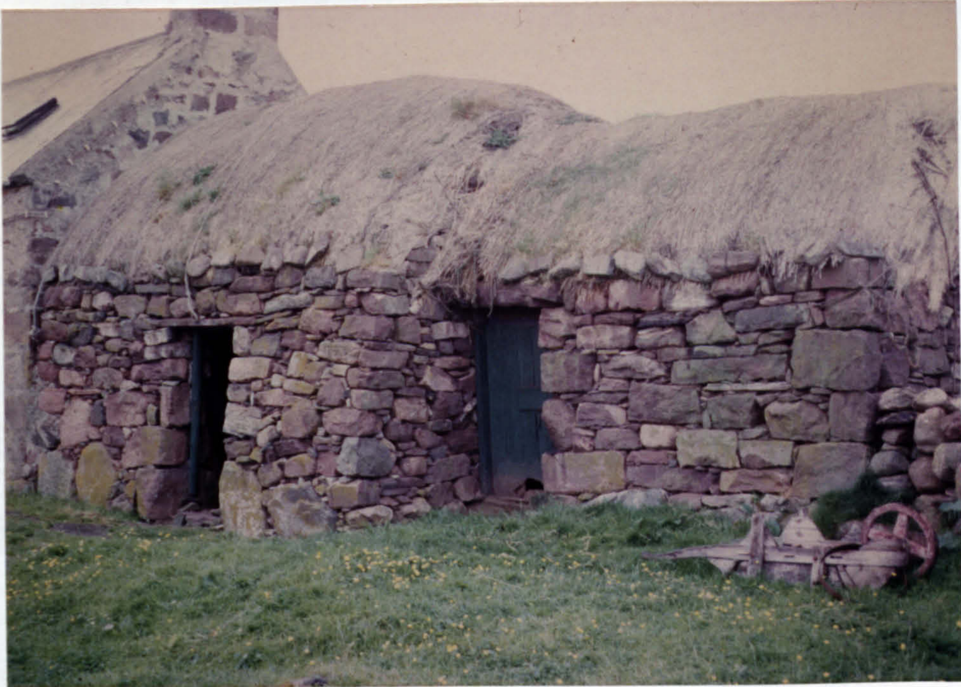
Plate 70. Old style of building on Balcladich (Bellachlattach) now used as byres or stores
