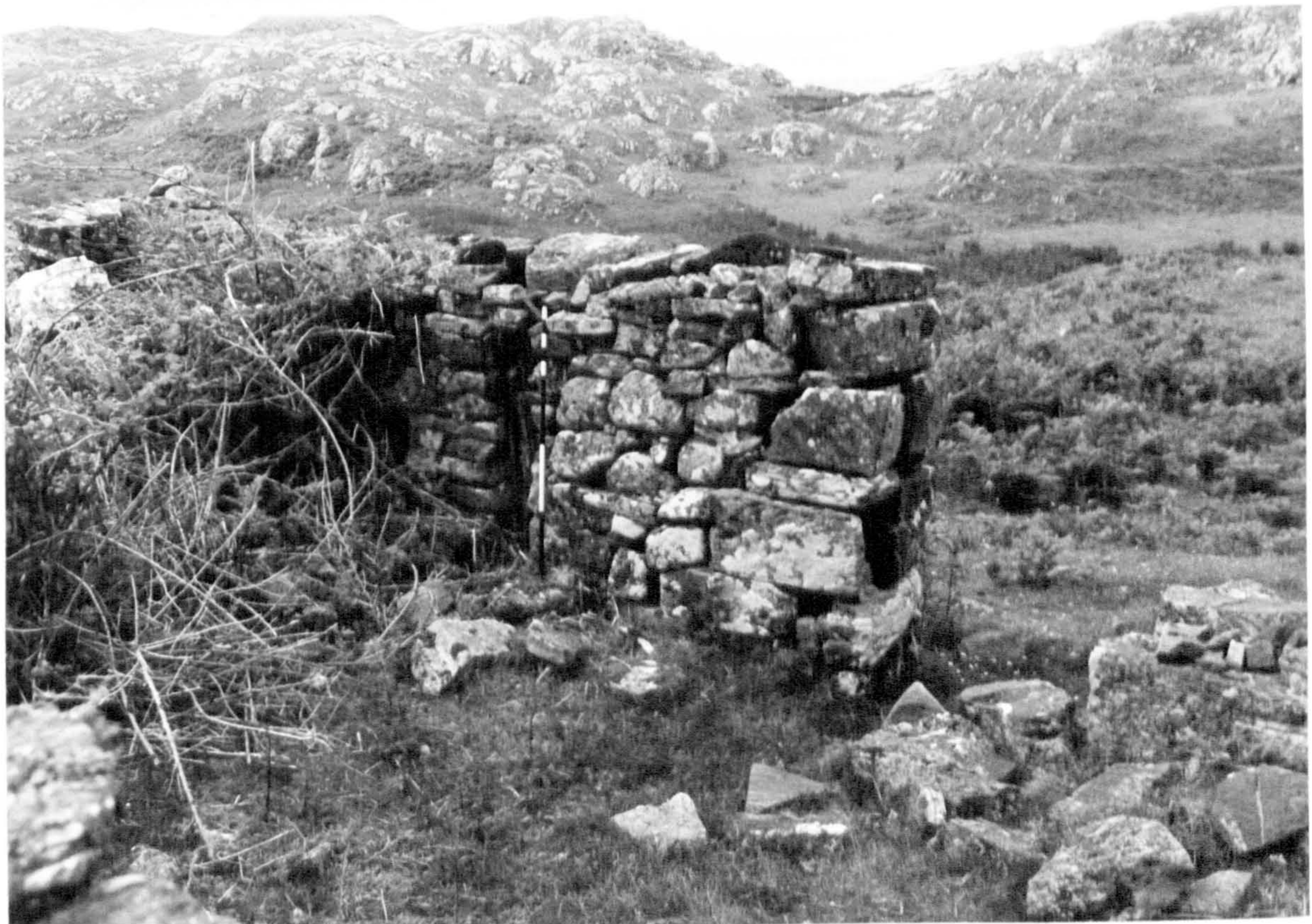
Plate 83. Interior of Building E, Glananter sheeling, showing cruck slot and doorway in NW wall (Figure 71).
