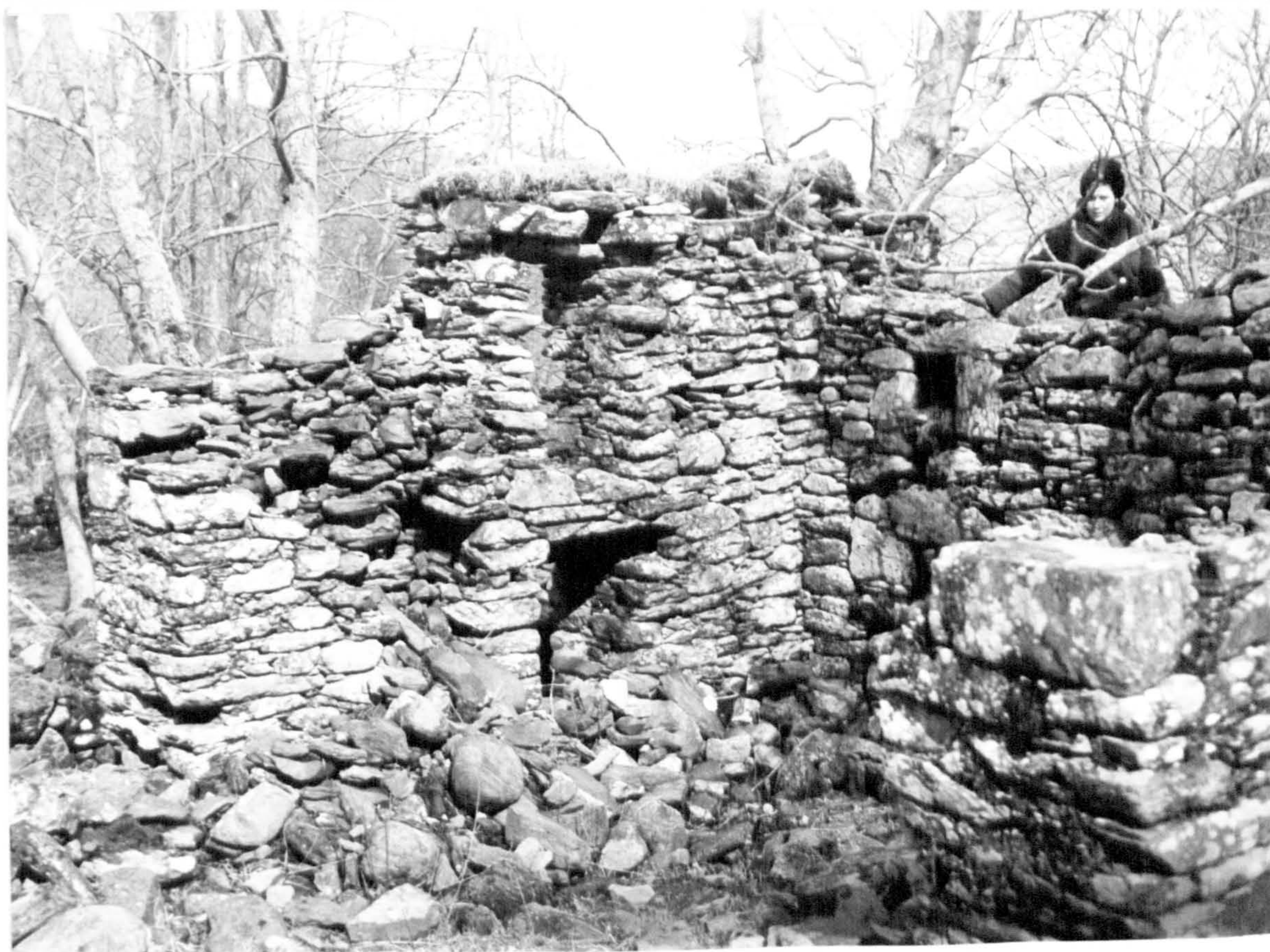
Plate 37. Lawers Mill, interior showing upper and lower windows
