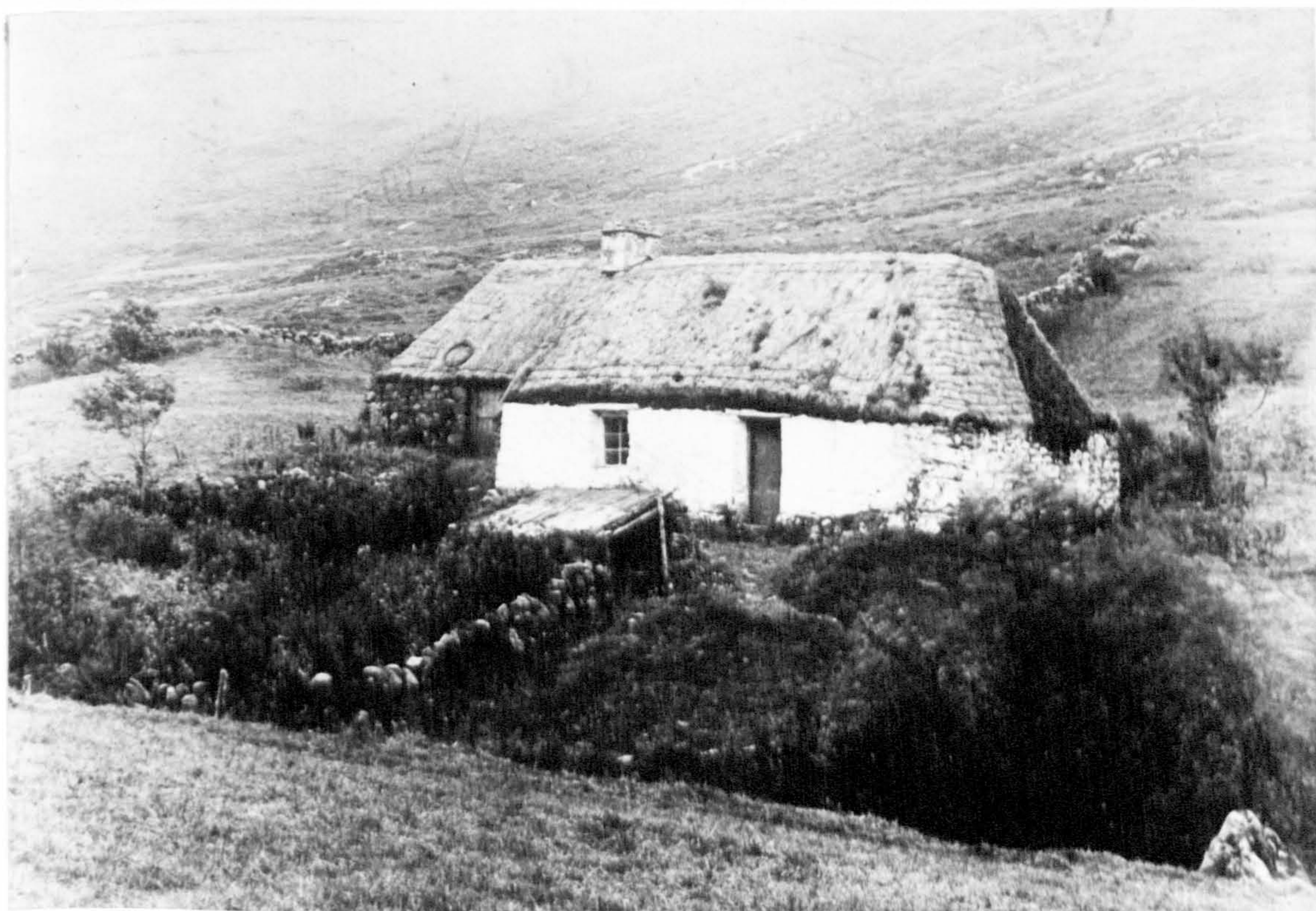
Plate 107. Building O at Auchindrain, c. 1886. One end hip-roofed.
