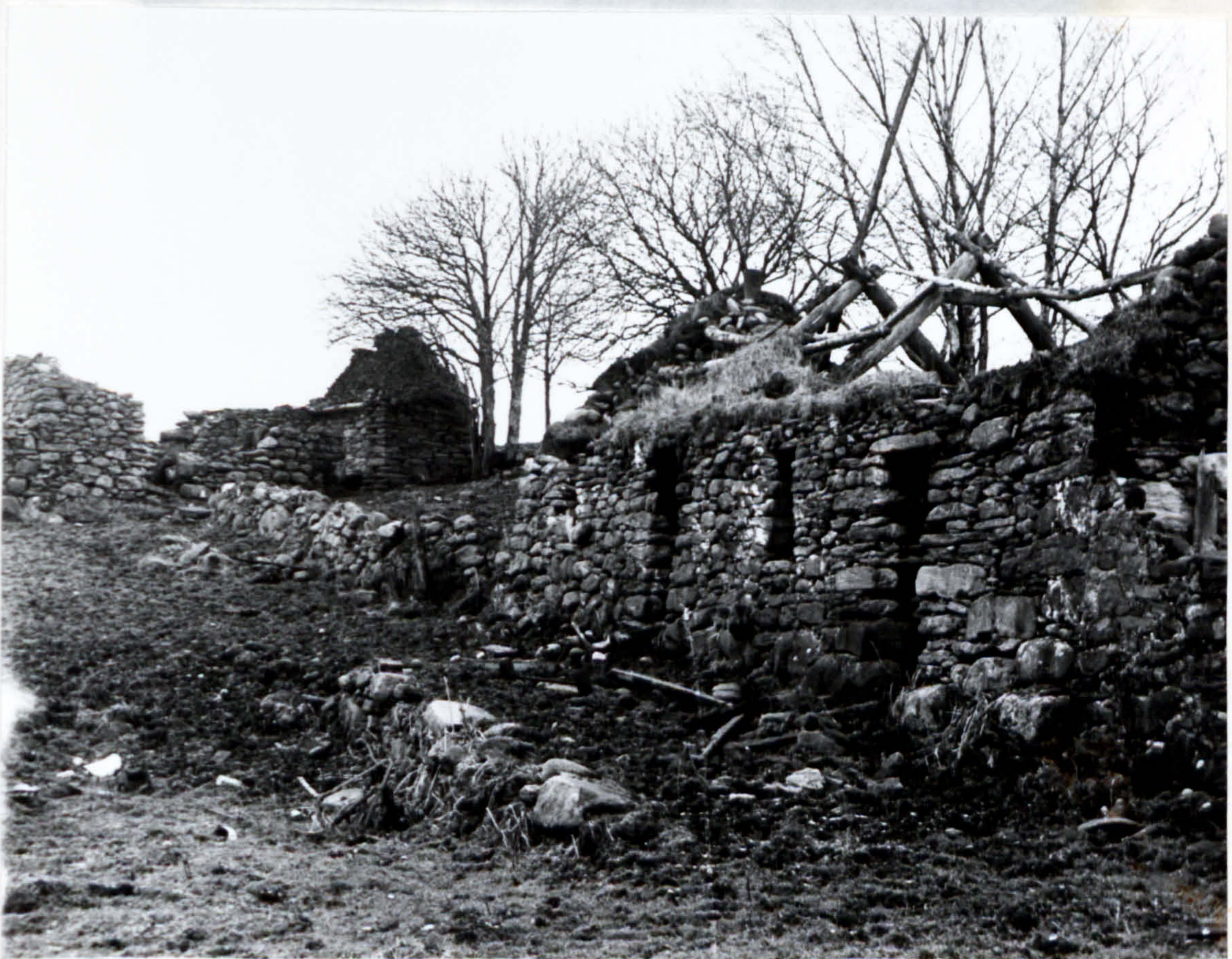
Plate 24. Building A in Cluster B on Cuiltrannich with Building B (latterly used as a smithy) in the background. (1966).
