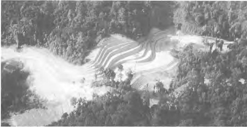
Figure 4. Pipeline and road construction have caused serious soil erosion problems along most of the 67 km of their routes, especially in primary, evergreen, forested areas. Photo: Scott Poynton, 9 March 1998.
