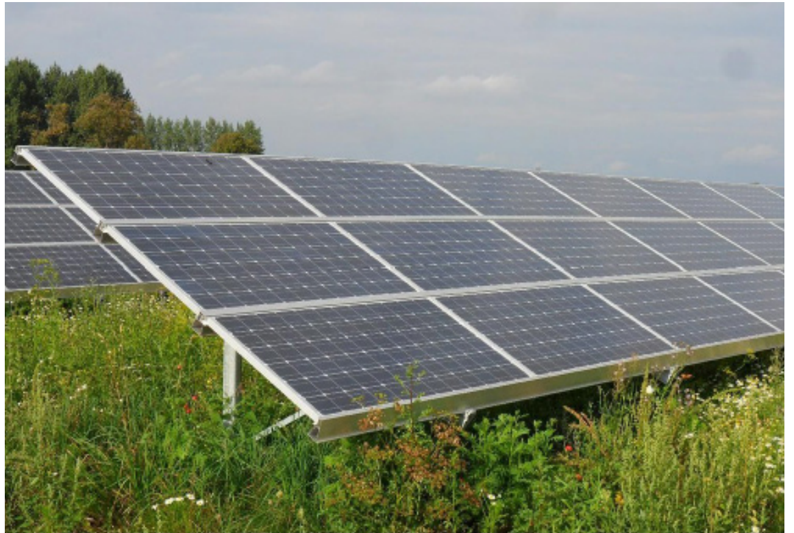
Courtesy of Thomas Kohler via Flickr Traditional photovoltaic cells generate between 150 and 200 watts per square meter, but they require sunlight to function.
