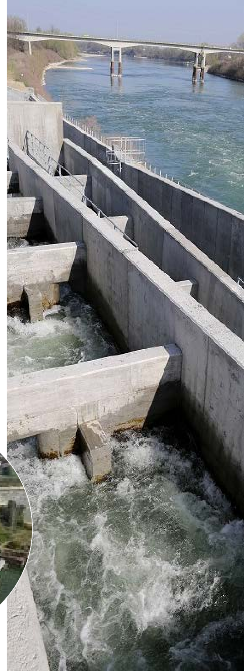
Fish passage at Isola Serafini Dam.
