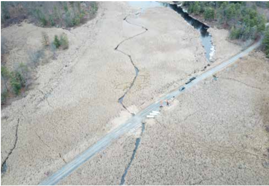
The causeway across the marsh prevented the historic water flow through the marsh, and allowed cattails to fill in.
