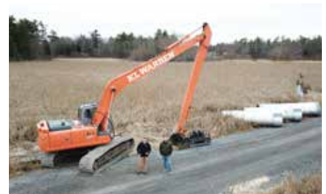
Culverts were installed under the causeway.
