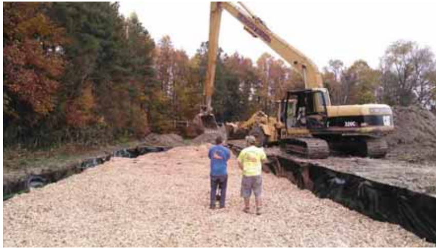
Figure 9: Denitrification Bioreactor example showing the subsurface woodchip-filled pit.
