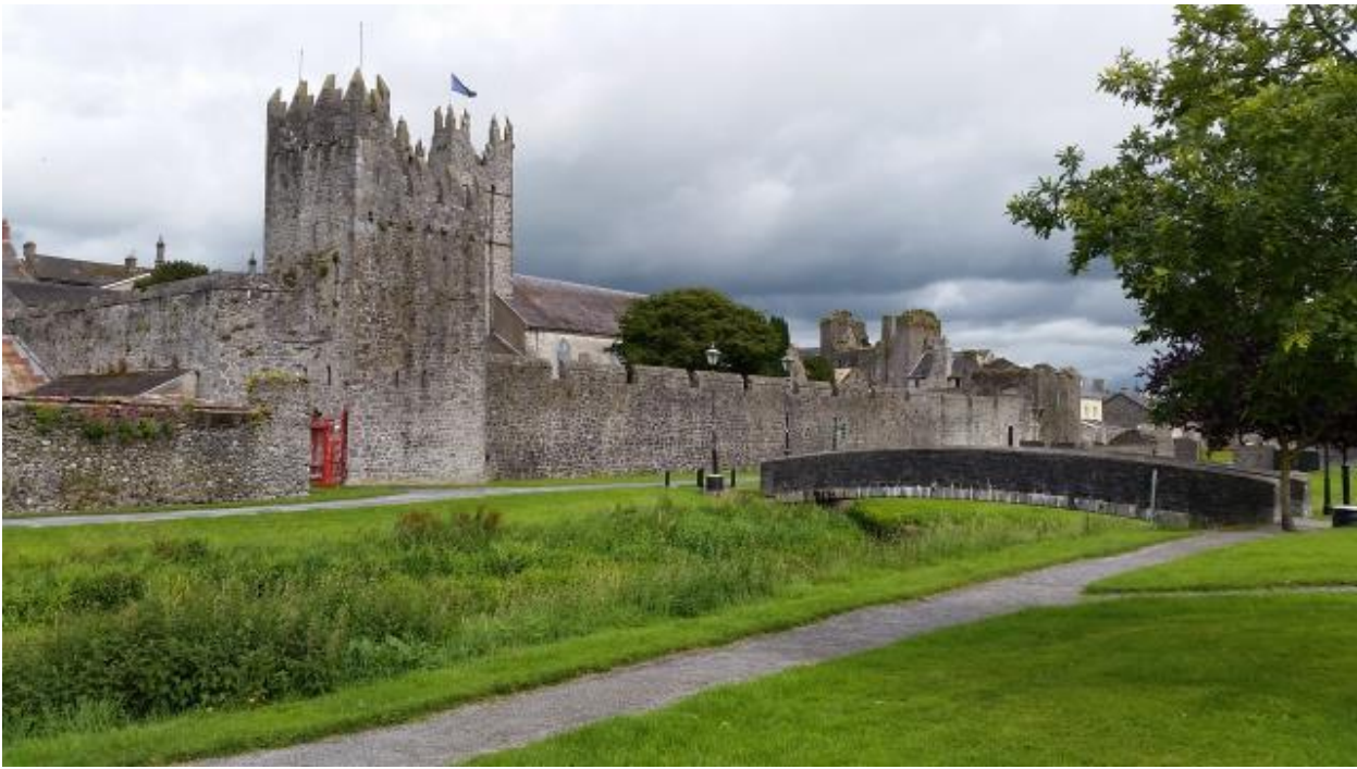
Figure 2.5 Anglo-Norman Structures in Fethard (Photo - Clare S Brindley)
